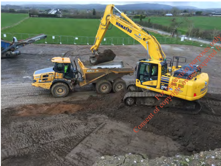
Figure 3-1: Typical Equipment Landfill Capping: Subsoil movement and placement
