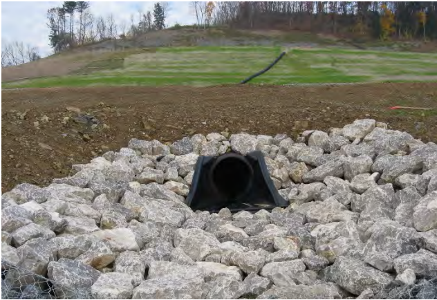
Figure 3-4: Typical Riprap Protection at Culvert Outfall
