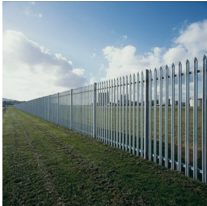
Figure 3-1: Typical Palisade Style Fencing 2
