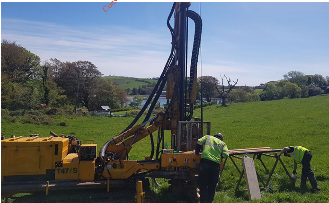
Figure 3-4: Typical Rotary Rig for Borehole Drilling
