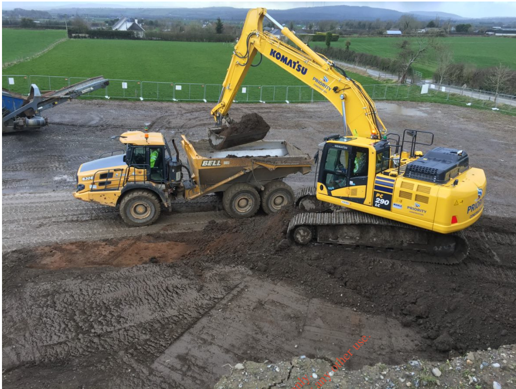
Figure 3-2: Typical Equipment Landfill Capping: Subsoil movement and placement
