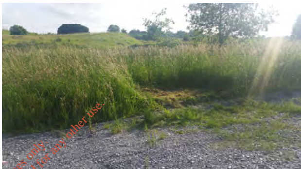
Photo 4. BH4 chamber top and setting
