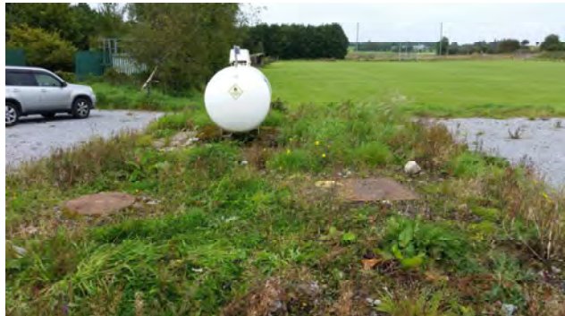
Photo 6. BH6 chamber on left and setting. Tank is a FloGas fuel tank, with gas piped to the community centre.
