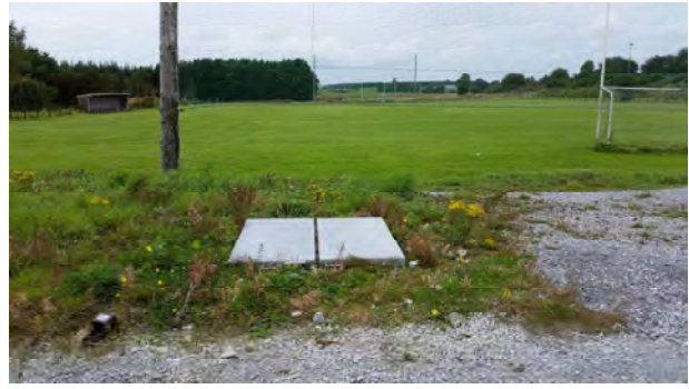
Photo 2. BH2 chamber top and setting
