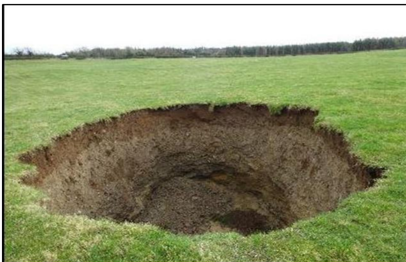
Figure 31: Main Fissure sinkhole approximately 13 m (long) x 8 m (wide) x 7 m (deep)
