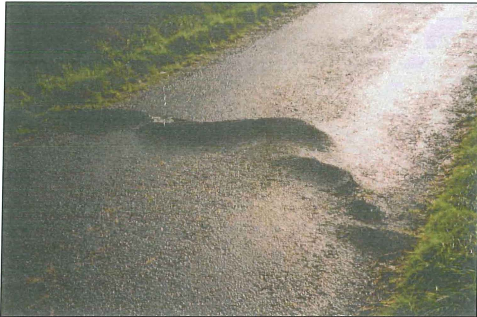
Photo 9. The central pressure ridge at the bottom of the hill, looking south, in early February.
