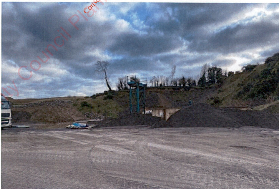
Image 2: South west corner of existing quarry
