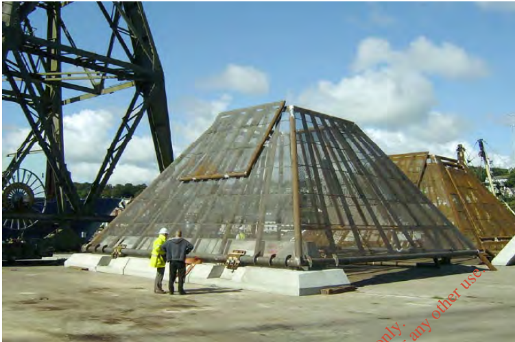
a) Wellhead protection structure
