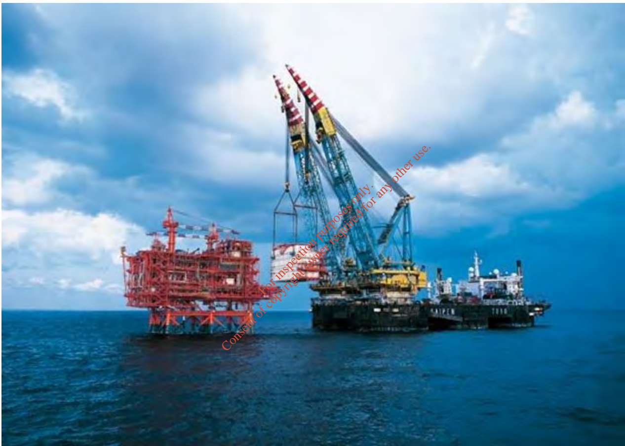
Figure 3.14: Conventional HLV, in this case Saipem 7000, lifting a topsides module
