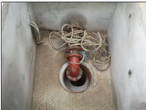
Photograph 3 PW1 showing the well head and the dry chamber during pumping (Nov 2011)
