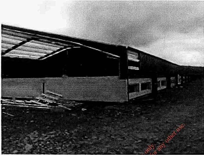
Close-up of planning ref. 20/416 under construction
