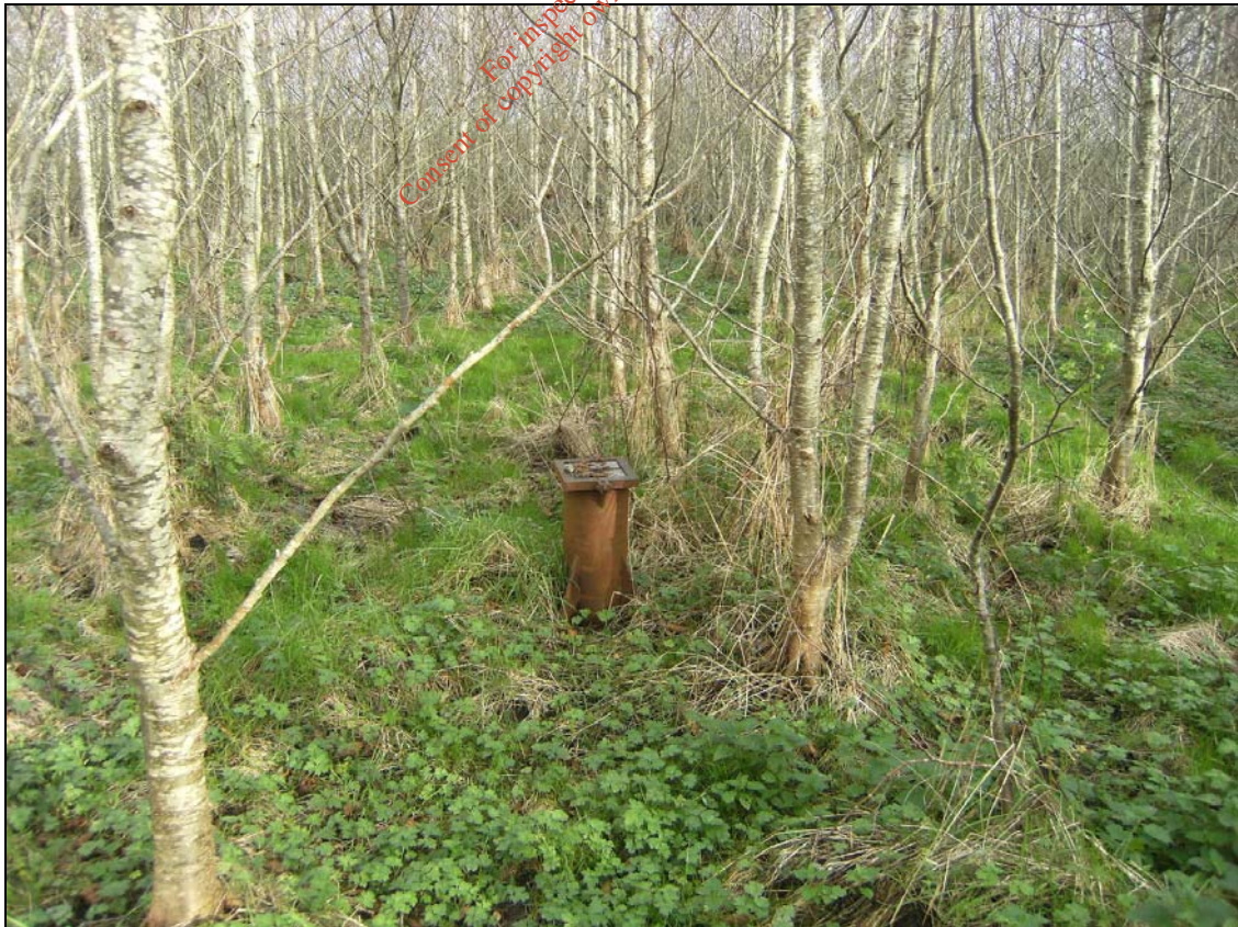
Photo No 2; Passive vent
