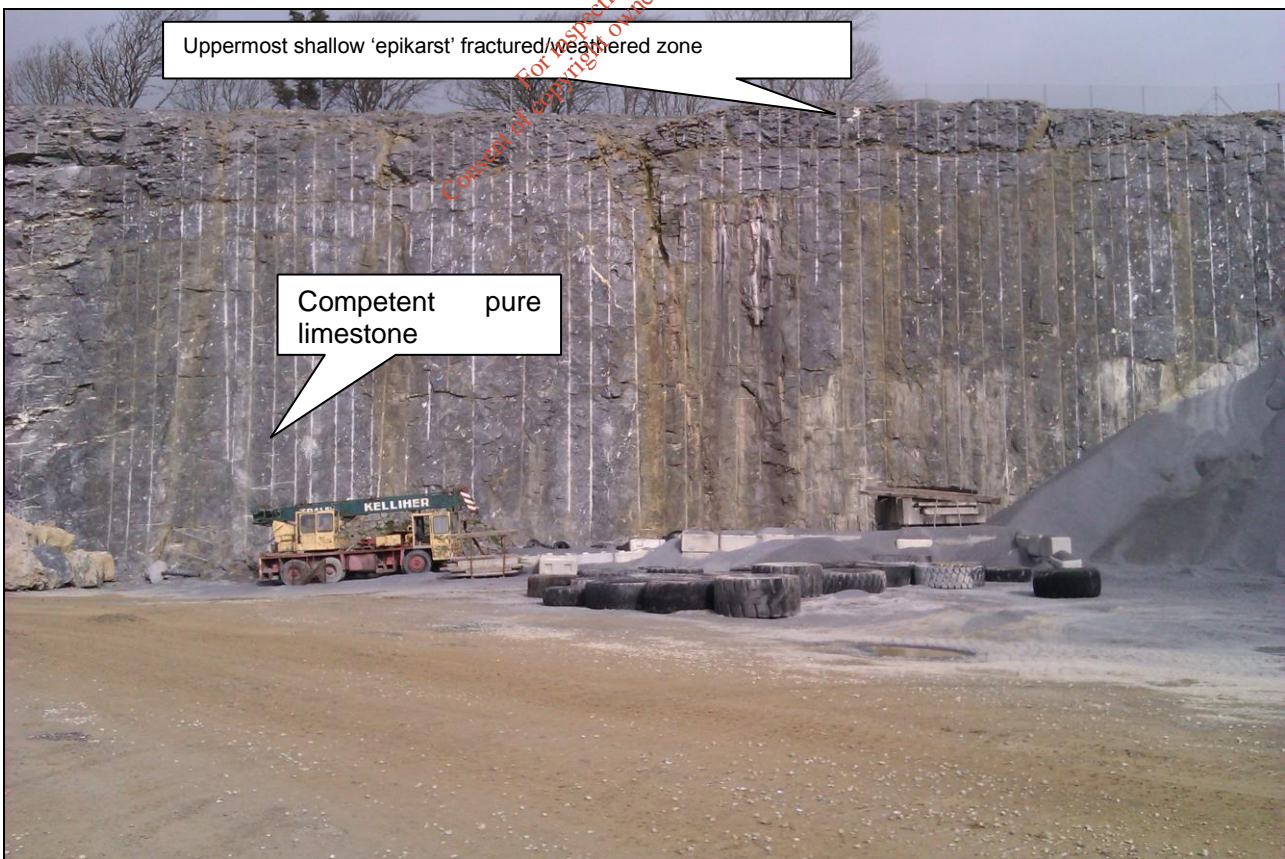
Photograph 7 East Quarry face
