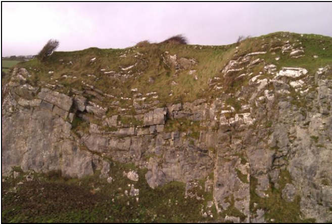
Photograph 11 Dirtoge Lst Fmn; upper most 2m indicate increased weathering and fracturing
