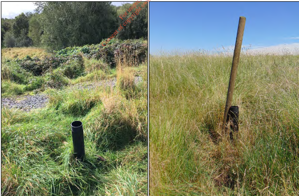
Figure 4.2: Leachate Monitoring Boreholes BH5 and BH6
