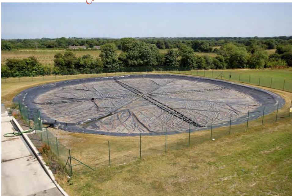
Plate 2-1: Covered Leachate Lagoon
