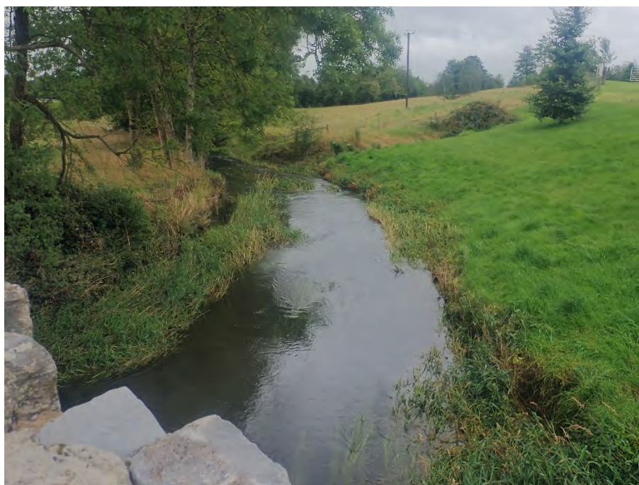
Plate 3.4 Representative image of site 3 on the River Nanny downstream of the R153 road bridge on 22 nd August 2019 during higher water levels.
