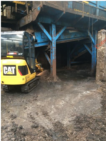
Plate 1: Removal of Screened material
