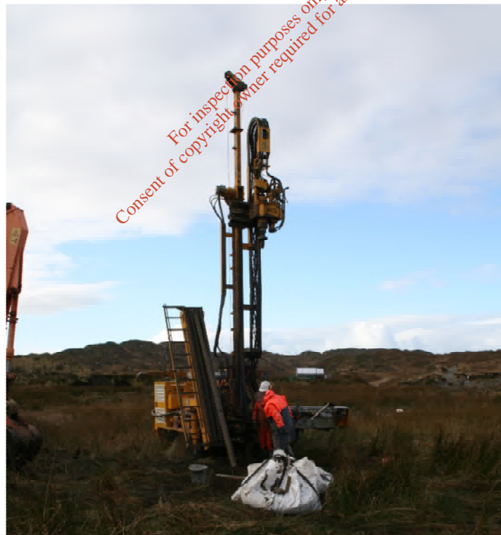
Plate 6: Drilling and installation of groundwater monitoring wells on former Clifden Landfill
