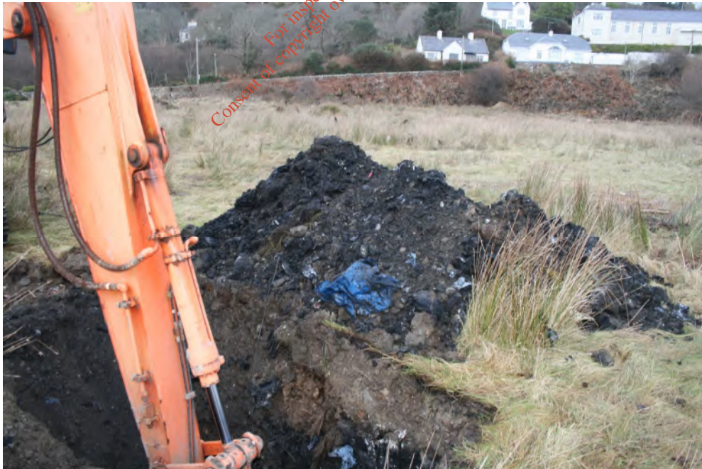
Plate 8. Supervision of Trialpit digging at Shore Road Landfill
