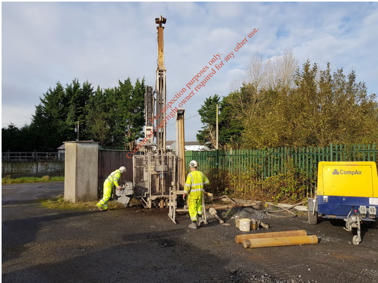
Plate 9. Drilling and installation of groundwater monitoring wells on former Ballygar Landfill
