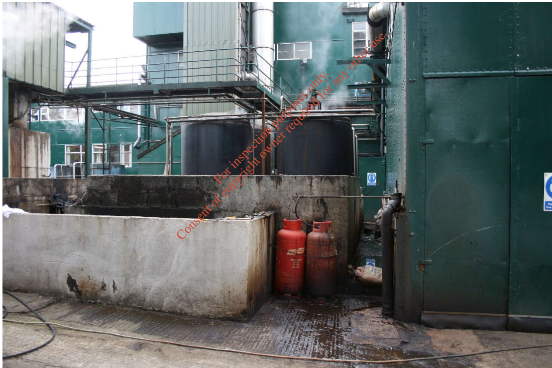
Plate 18: Cooley Distillery Historic Waste Landfill Investigation
