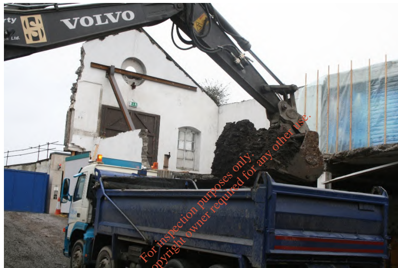
Plate 11. Supervision of removal of hydrocarbon contaminated soil from basement area.
