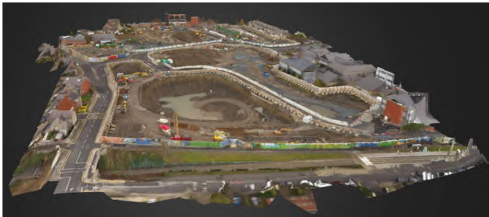
3D Model of NCH/St. James Hospital construction site (2 nd January, 2018)
