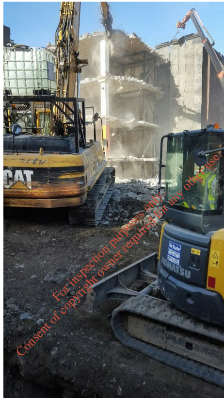
Plate 13. On-going demolition during site investigation of Clanwilliam Site.
