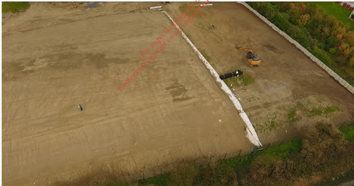
Plate 7. Drone aerial photo of landfill cap construction in October, 2020.
