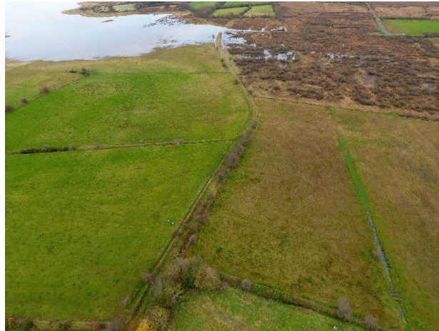
4K Aerial drone photo of SAC adjacent to historic landfill
