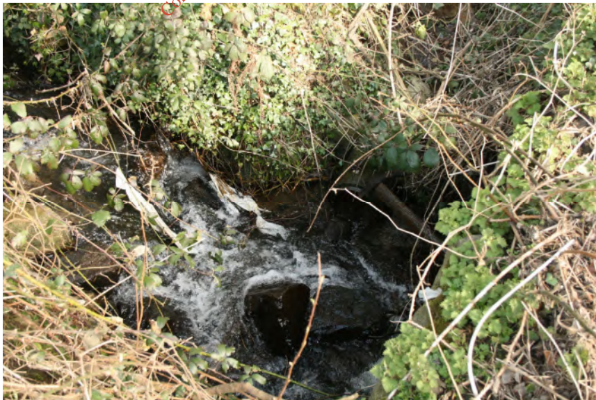
Plate 9. Surface Water Monitoring point located beside former landfill in Dundalk
