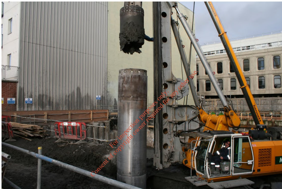
Plate 14. Secant piling along periphery of new basement at RCSI Site.
