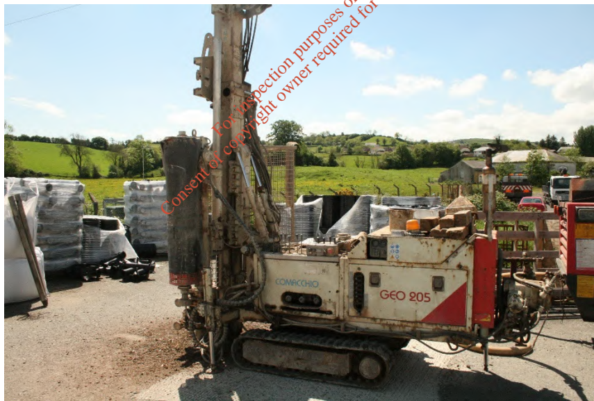
Plate 10. Drilling and installation of groundwater monitoring wells on UBP brownfield site.
