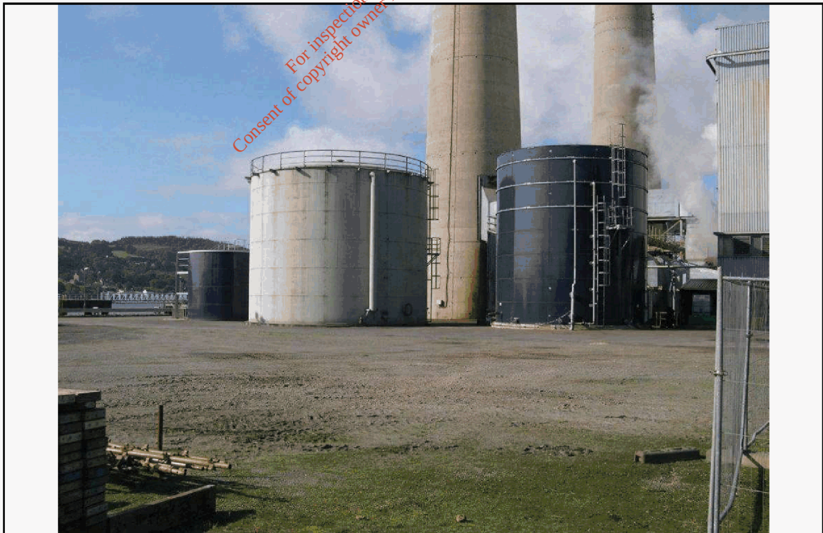
Location No: 6 View west towards chimneys.
