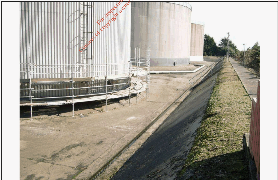
Location No: 20 View east along tank farm.
