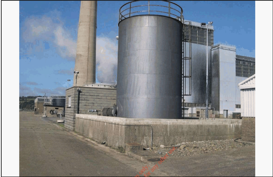
Location No: 4 Stripping Tank.
