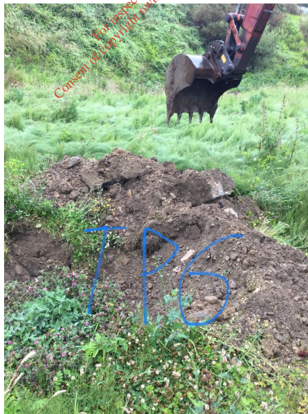
Plate A1.12 Photograph of stockpile of material in TP6
