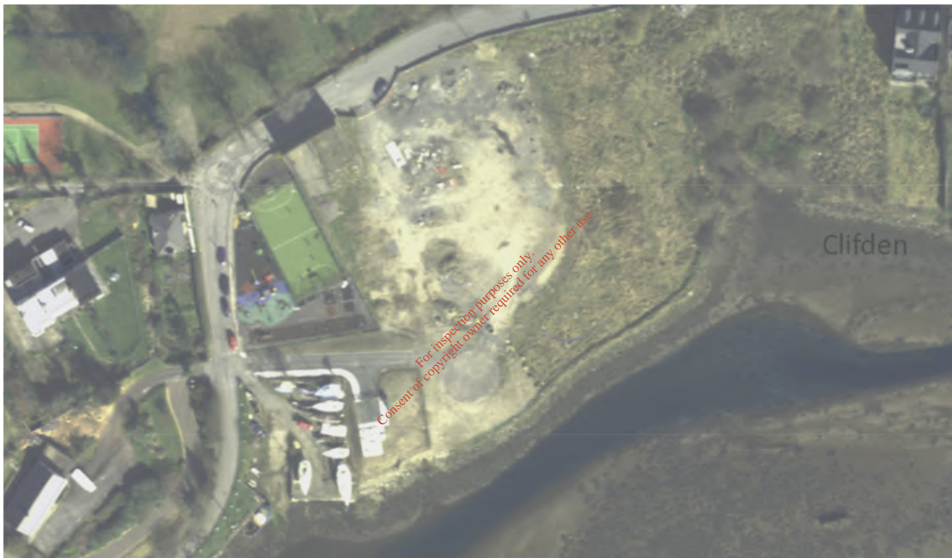
AERIAL PHOTOGRAPH TAKEN FROM ORDNANCE SURVEY IRELAND SHOWING SITE BEFORE THE DEMOLITION OF THE HANDBALL ALLEY (POSSIBLY TAKEN IN LATE 2017). GROUNDWORKS ON THE INSTALLATION OF NEW SEWERAGE DRAINAGE INFRASTRUCTURE IS VISIBLE.
