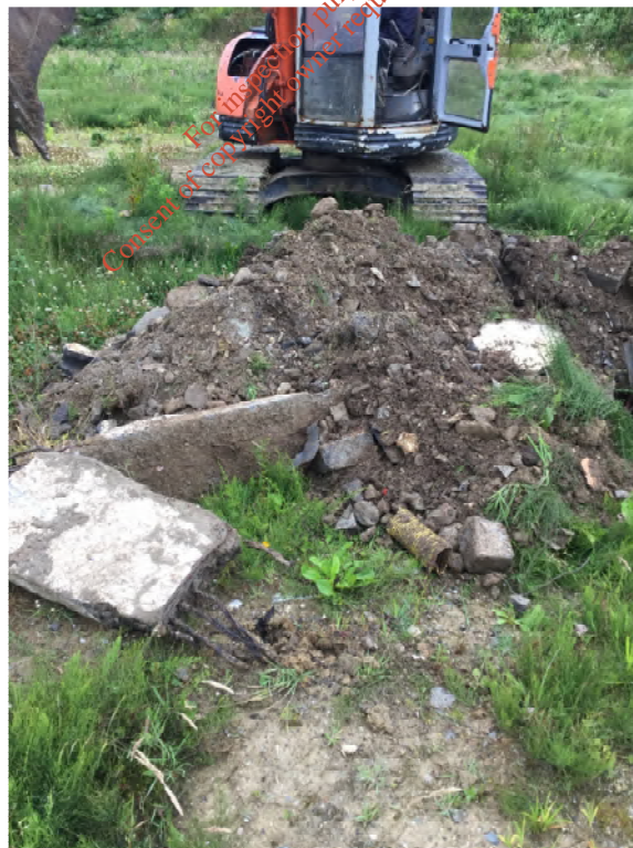
Plate A1.14 Photograph of stockpile of material in TP7
