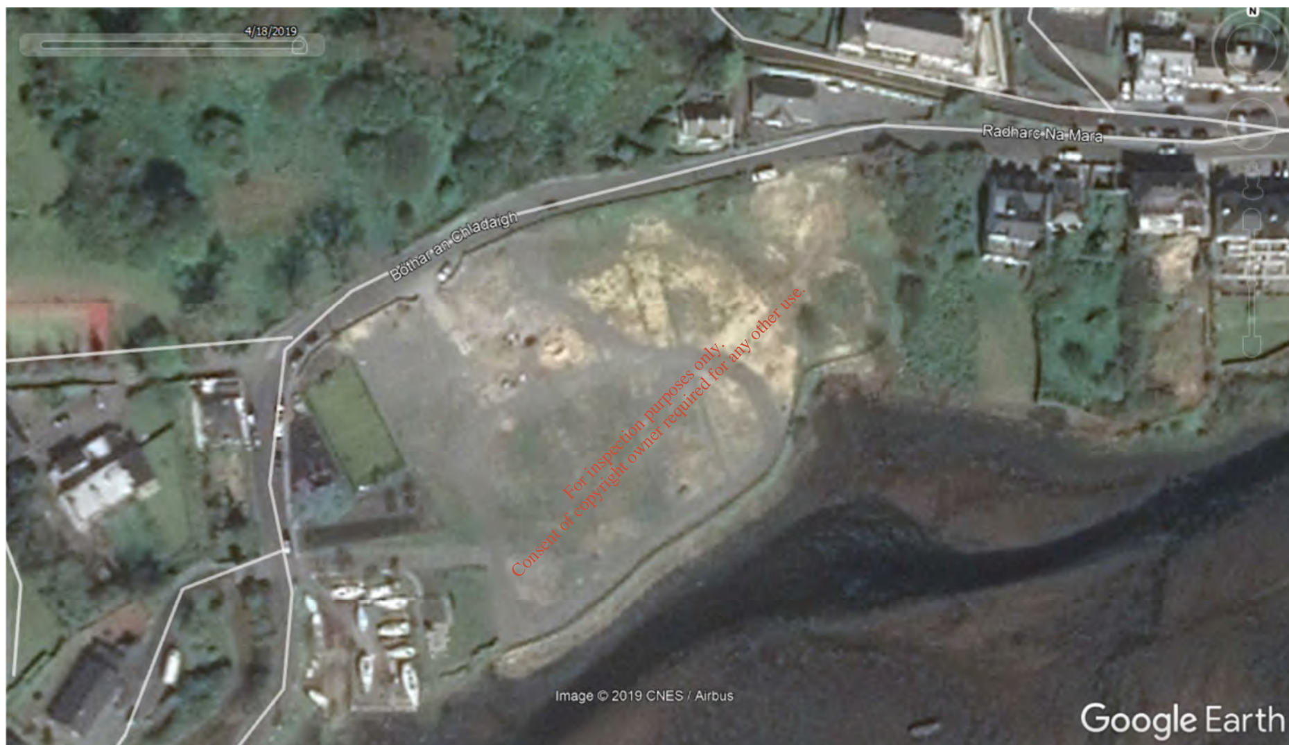
AERIAL PHOTOGRAPH TAKEN FROM GOOGLE EARTH SHOWING SITE AFTER THE DEMOLITION OF THE HANDBALL ALLEY, THE IMPORTATION OF C&D WASTE AND THE INSTALLATION OF THE 5 LAND DRAINS (MOST LIKELY TAKEN IN 2019)
