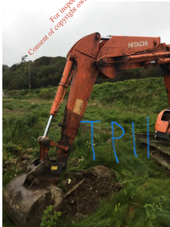
Plate A1.22 Photograph of stockpile of material in TP11
