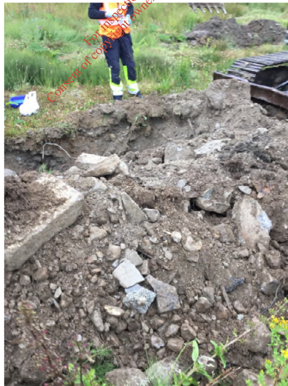
Plate A1.10 Photograph of stockpile of material in TP5
