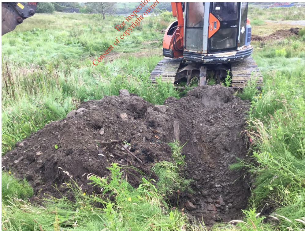
Plate A1.18 Photograph of stockpile of material in TP9
