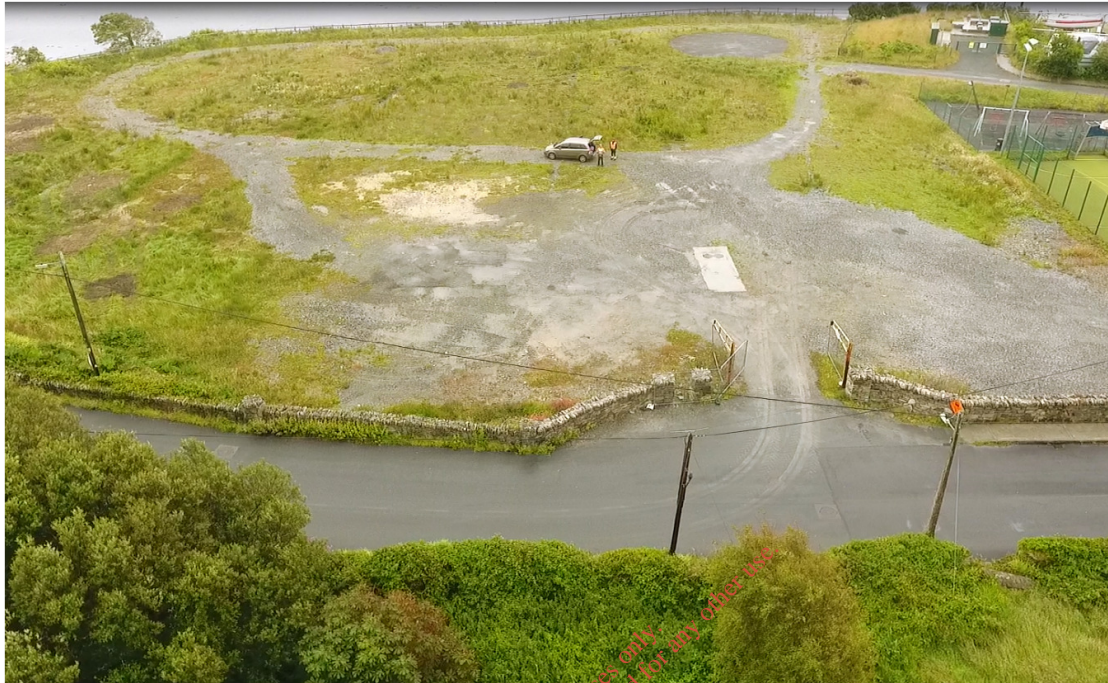
Plate 15. Aerial photograph taken at 30m elevation showing access manholes to foul sewer on concrete slabbing opposite site entrance.
