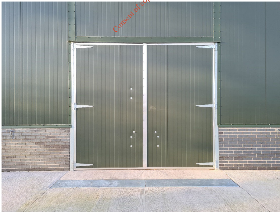
Plate 2. Photo of grated channel to the front of the existing poultry unit onsite.
