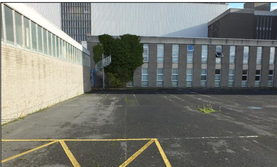
Figure 7.2: Poolbeg BESS Site
