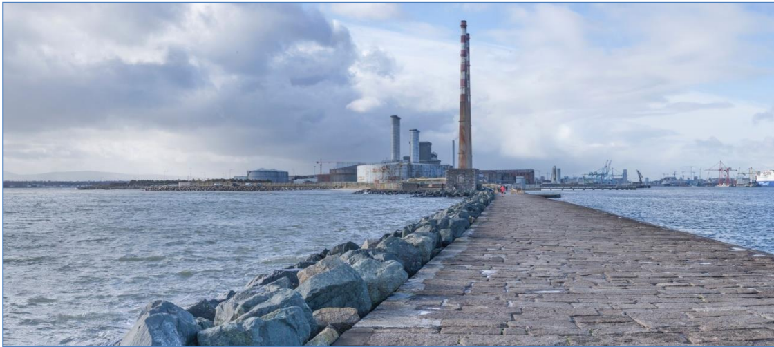
Figure 10.3: View of the Poolbeg peninsula from the Great South Wall/South Bull Wall
