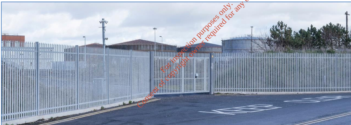
Figure 10.6: Vehicular entrance to the southwest of the site
