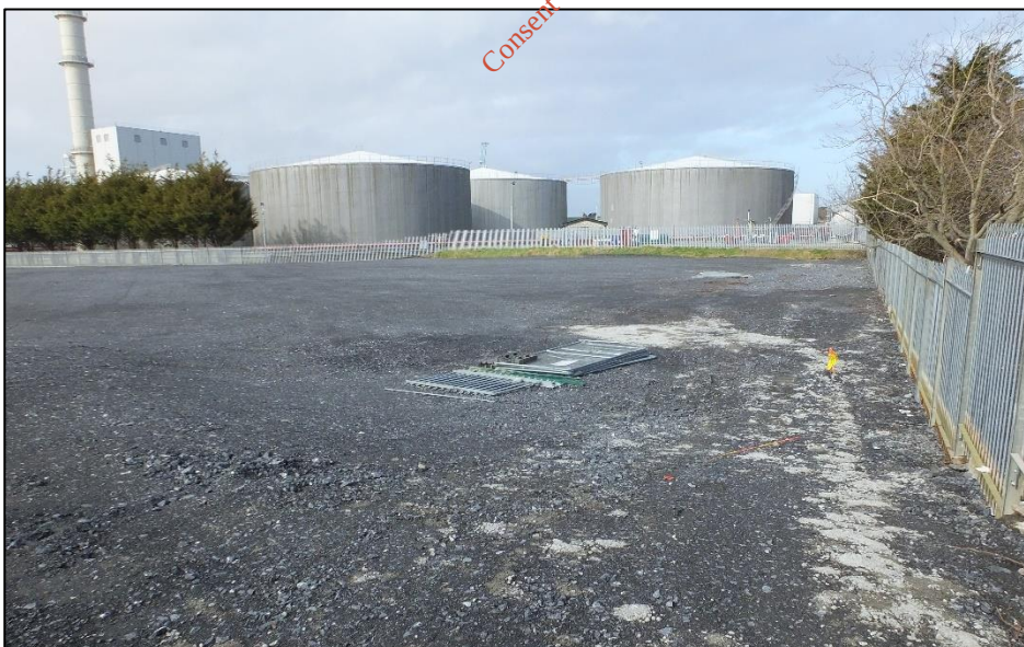
Figure 7.3: South Wall BESS Site
