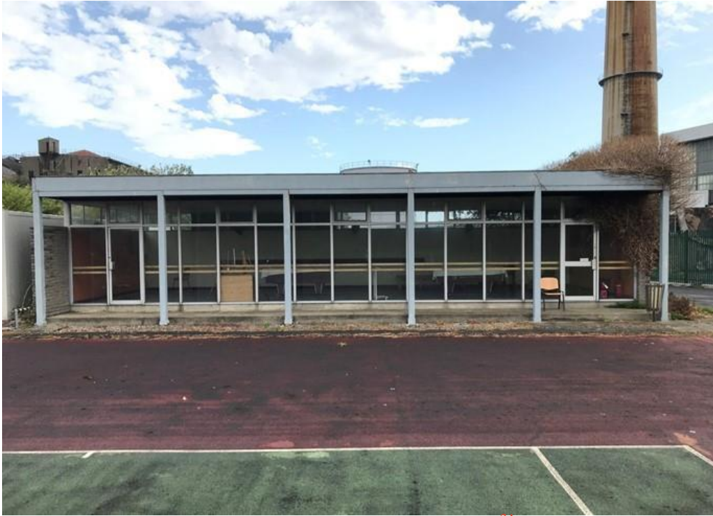
Plate 2: Safety Centre – southern elevation
