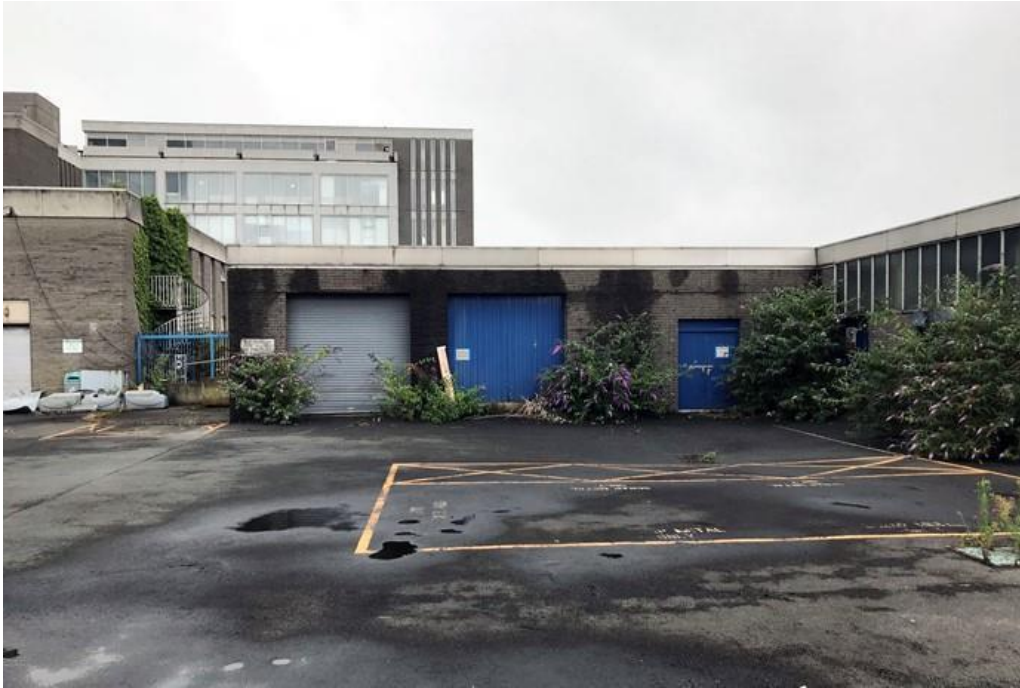
Plate 5: Store/workshop – northern elevation of wing
