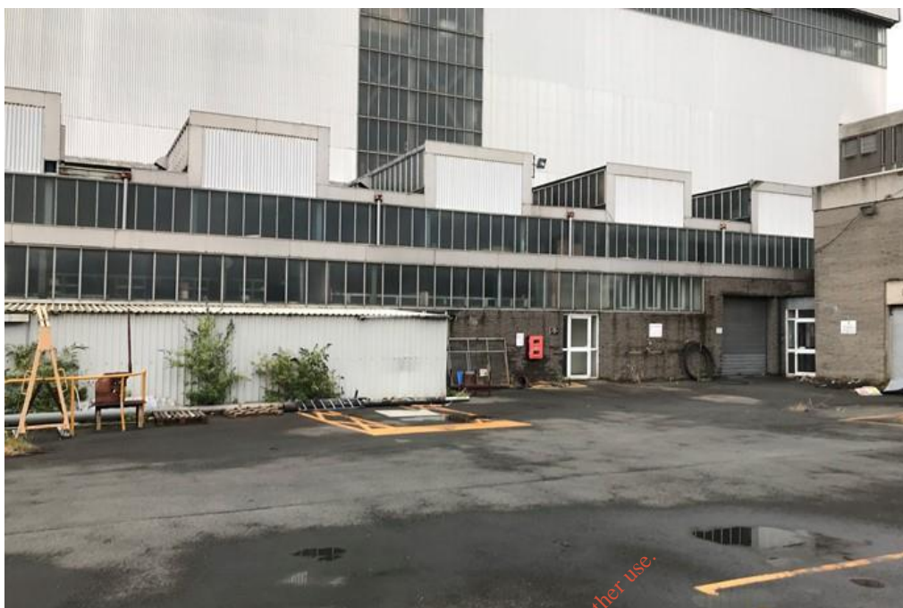
Plate 7: Main store/workshop with generating hall at rear
