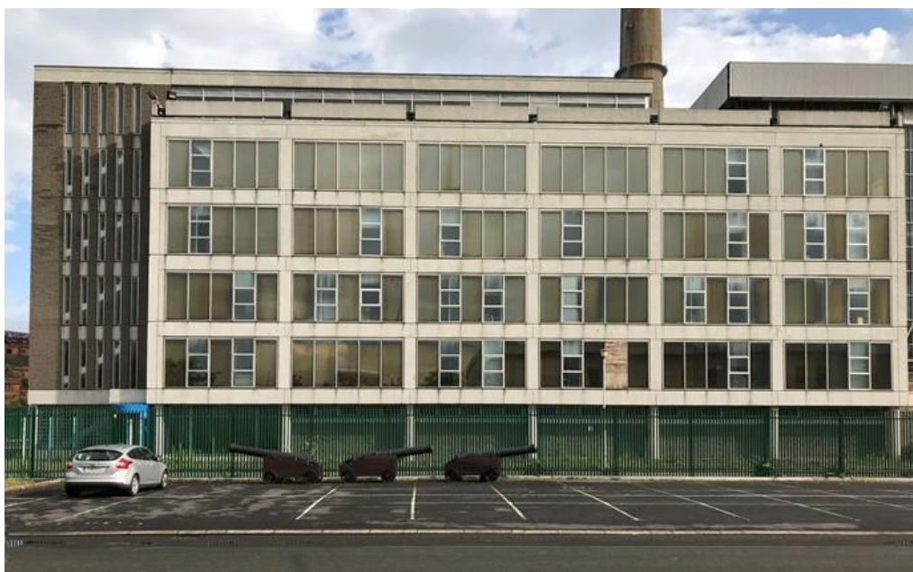
Plate 10: Administration building – southern elevation
