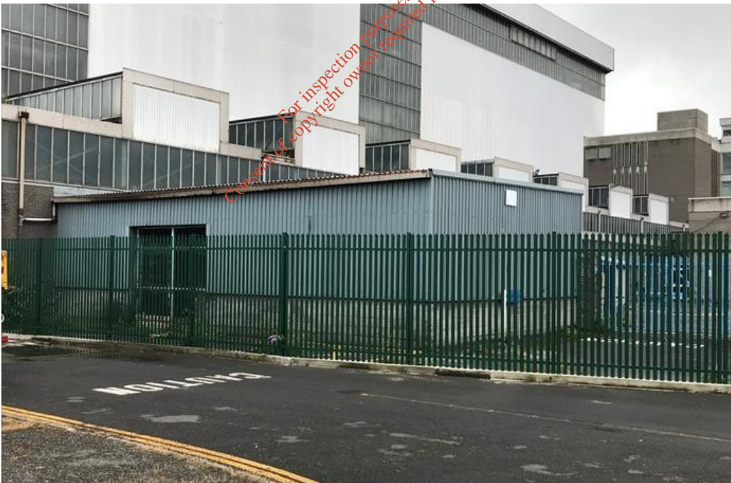
Plate 9: Main workshop/stores – single-storey wing at northern end
