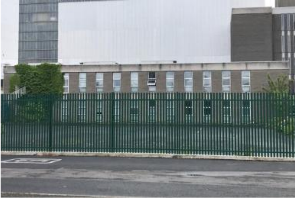
Plate 8: Main stores/workshop – two-storey section
