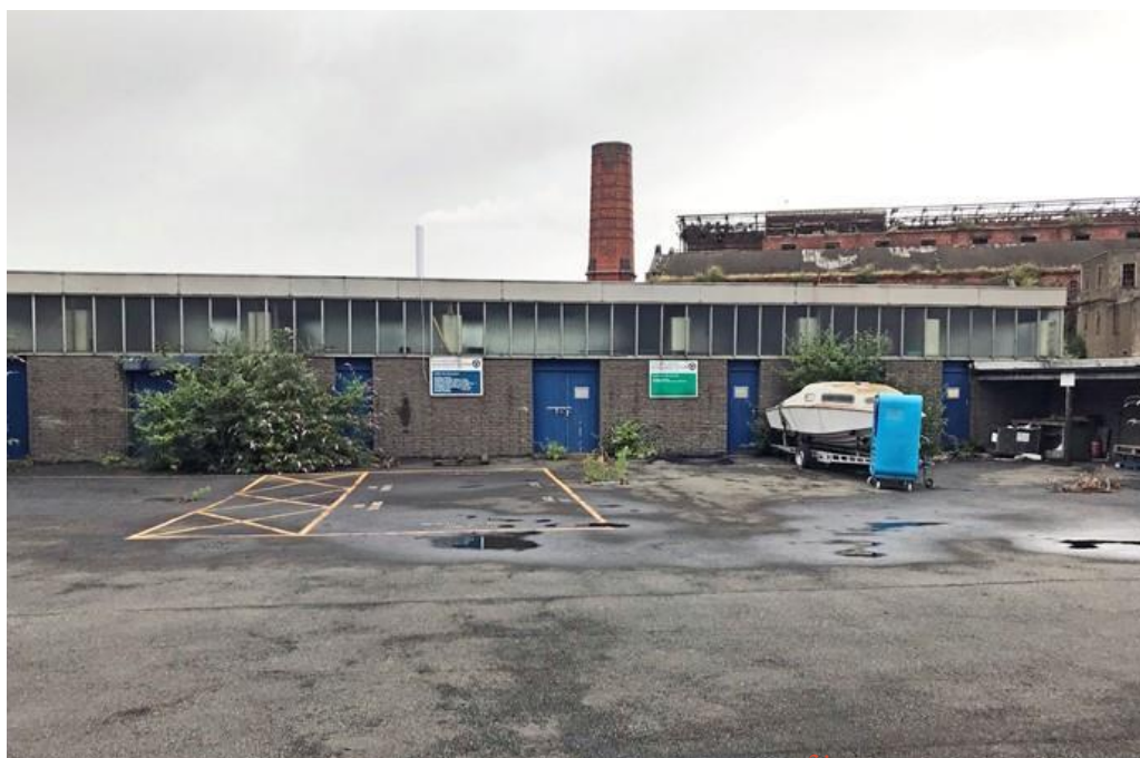
Plate 4: Store/workshop – eastern elevation
