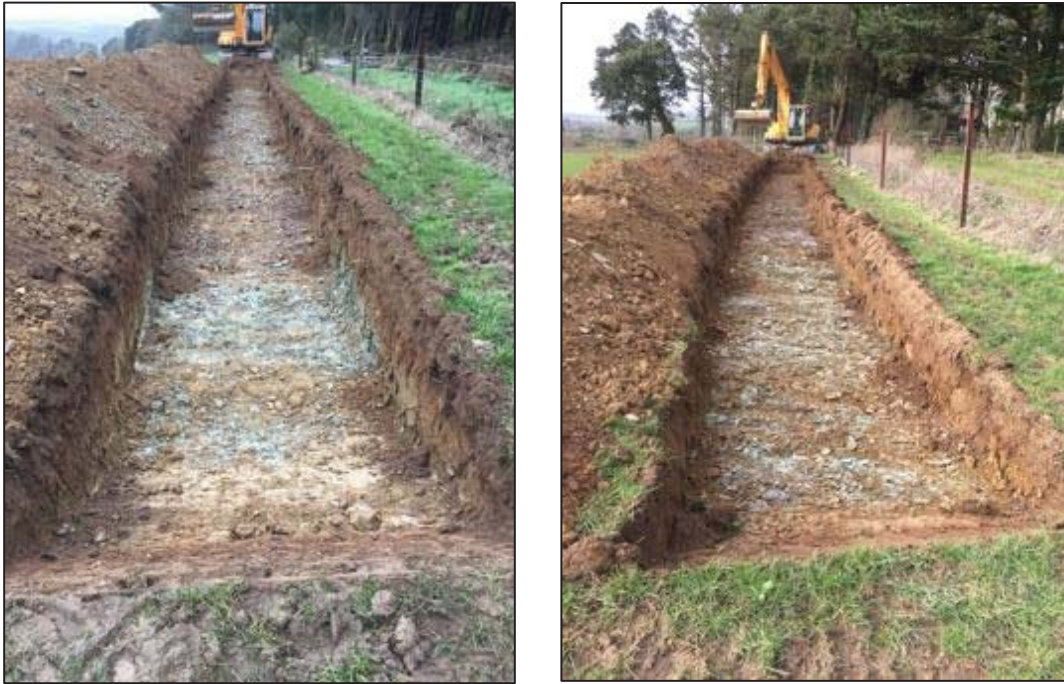
Plates 10 & 11: View of trenches 8 and 9 from the east, after excavation.
