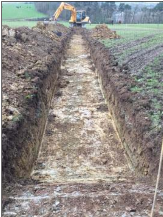
Plate 6: View of trench 4, from the east.
