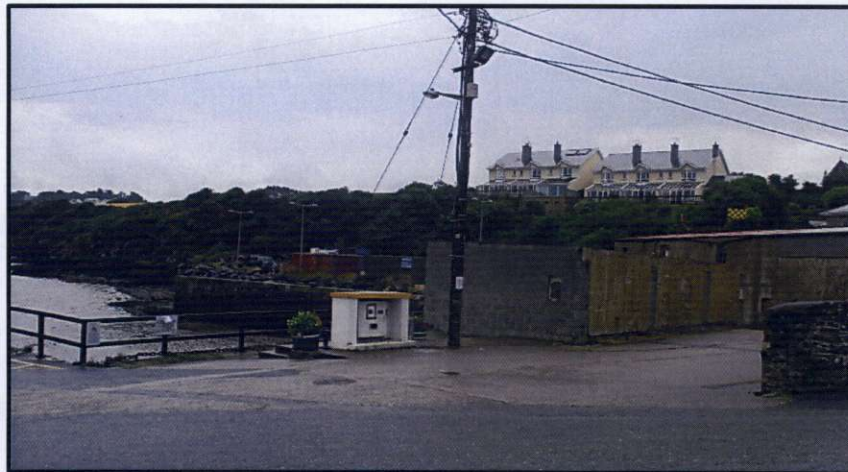
Location for Duncannon pumping station
