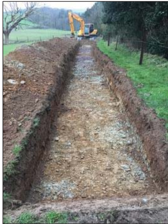
Plate 7: View of trench 5 from the east.
