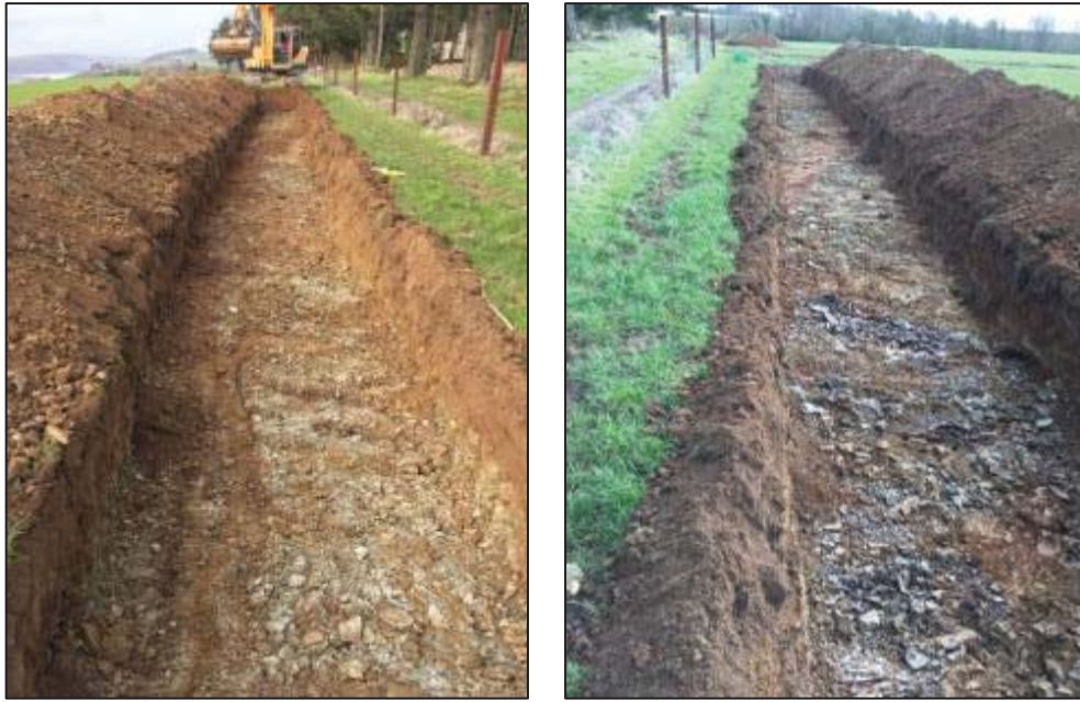
Plates 12 & 13: View of cut features in trenches 10 and 11.
