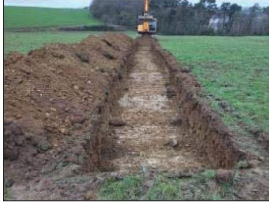
Plate 4: View of trench 3 from the east.
