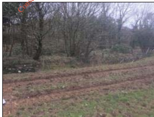
Plate 5: Detail of break in the wall, to the north of trench 4, from the south east.
