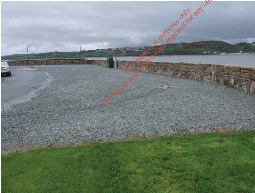
Figure 2.4: Site of pumping station at Arthurstown
