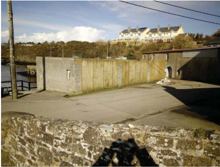
Figure 2.5: Site of pumping station at Duncannon
