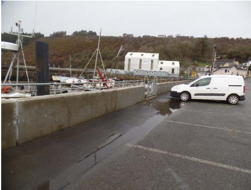
Figure 2.3: Site of pumping station at Ballyhack
