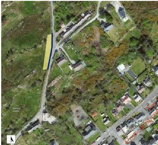
Figure 11 Habitat map offline area Foildarrig. Yellow – Scrub WS1, Dark blue - Stonewall and other stonework BL1
