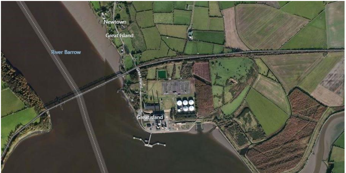
Figure 1: An aerial photograph showing the power station at Great Island, County Wexford.
