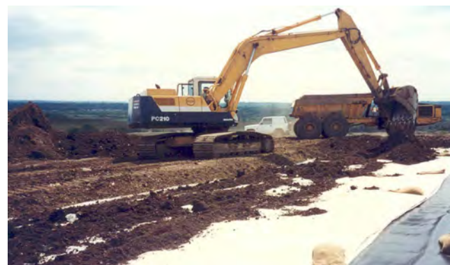
Fig. 8: First layer of covering
