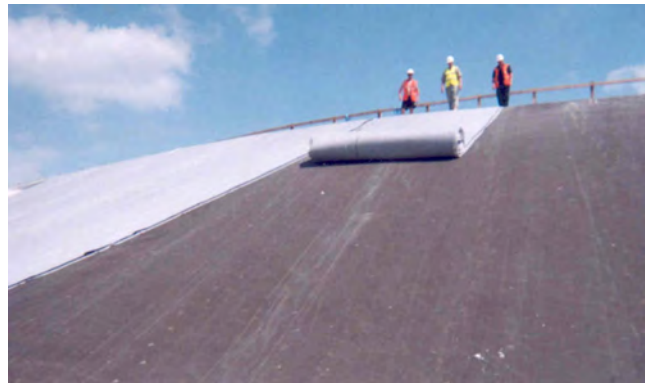
Fig. 5: Pozidrain being rolled downhill
