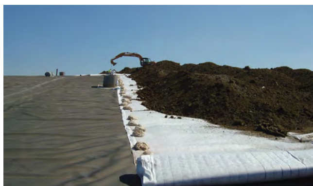
Fig. 4: Sandbags holding edges of Pozidrain in place
