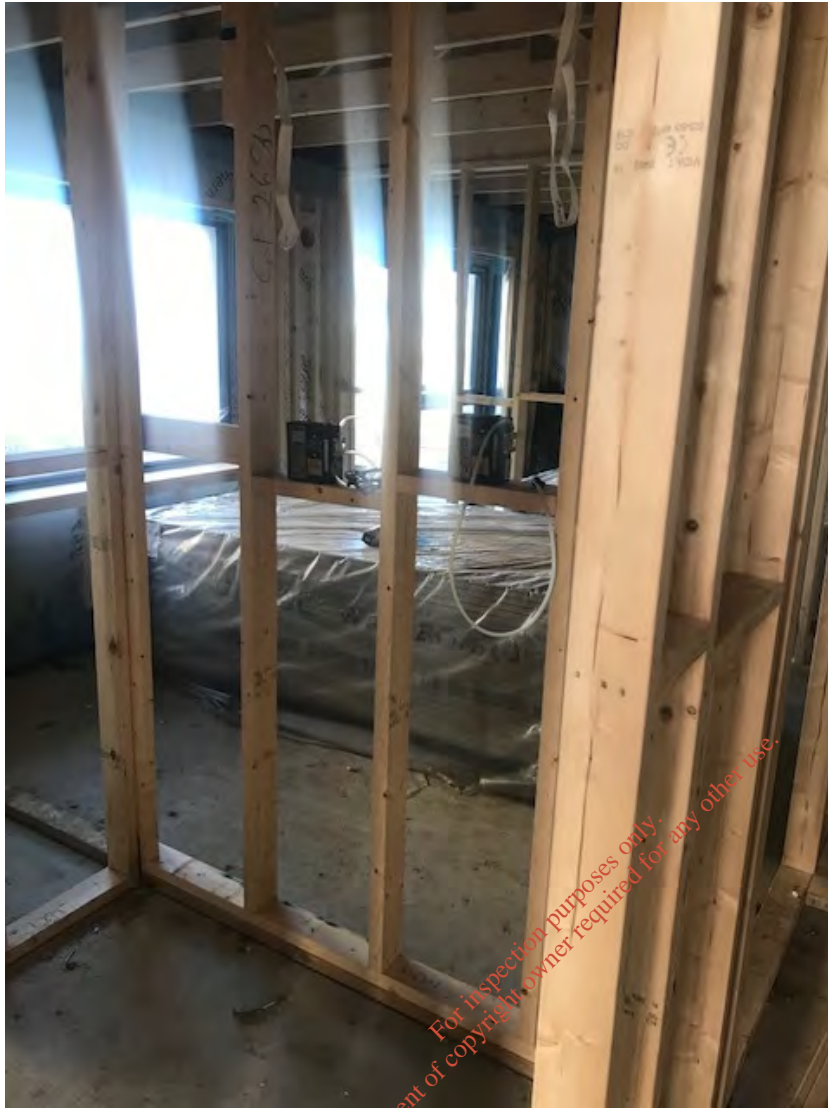
Figure 7.3. Location of monitoring in Hse 52
