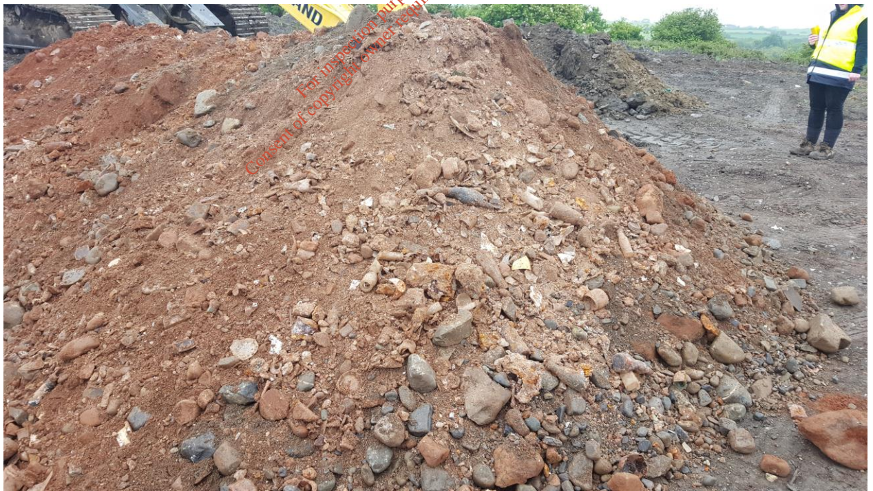
Plate A7.4 Photograph of stockpile of excavated soil and waste from TP5
