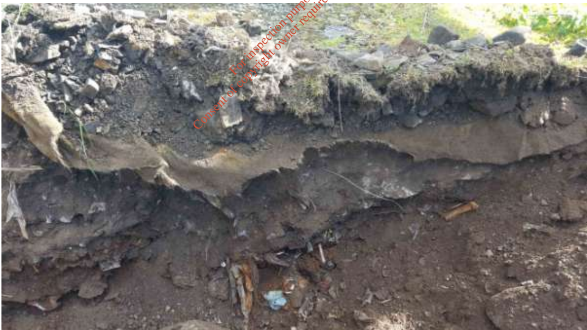
Plate 4. South facing section showing the modern fill, overlain by a geotextile membrane in turn overlain by the remains of the gravel track.
