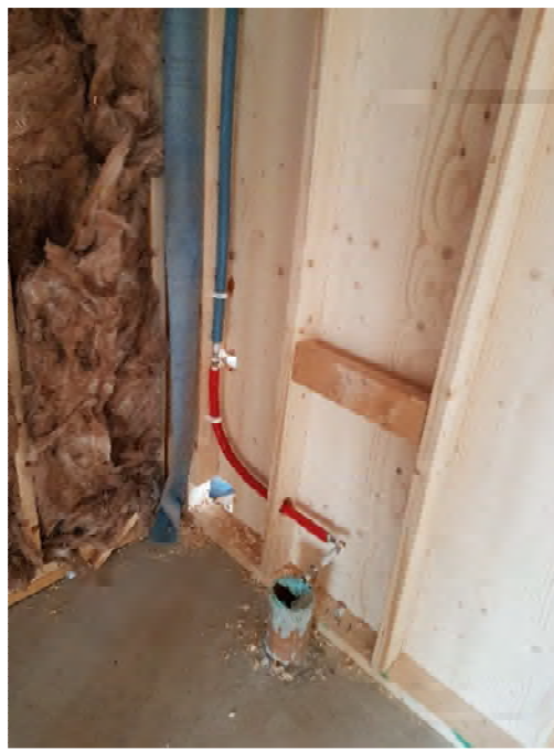
Plate 9. Services within newly built residences which were inspected and checked for the presence of landfill gases
