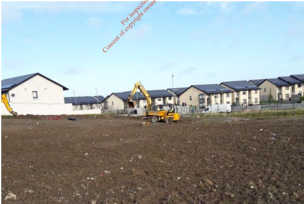
Figure 2.4 Regrading and Soil Spreading at Barnageeragh Landfill, October 2019
