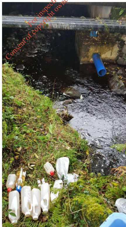
Plate 23. Photographs of SW5 surface water sampling area (note discharge pipe equipped with valve and services running in line with road)
