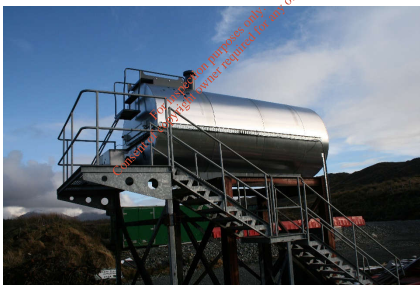
Plate 4. View of 10,000l aboveground storage tank used for the storage of road bitumen
