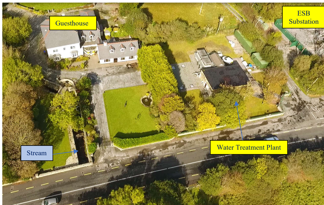
Plate 8. Galway County Council/Irish Water - Water Treatment plant located at corner of country road and national road N59 (note guesthouse to west of plant and ESB substation to east of site)
