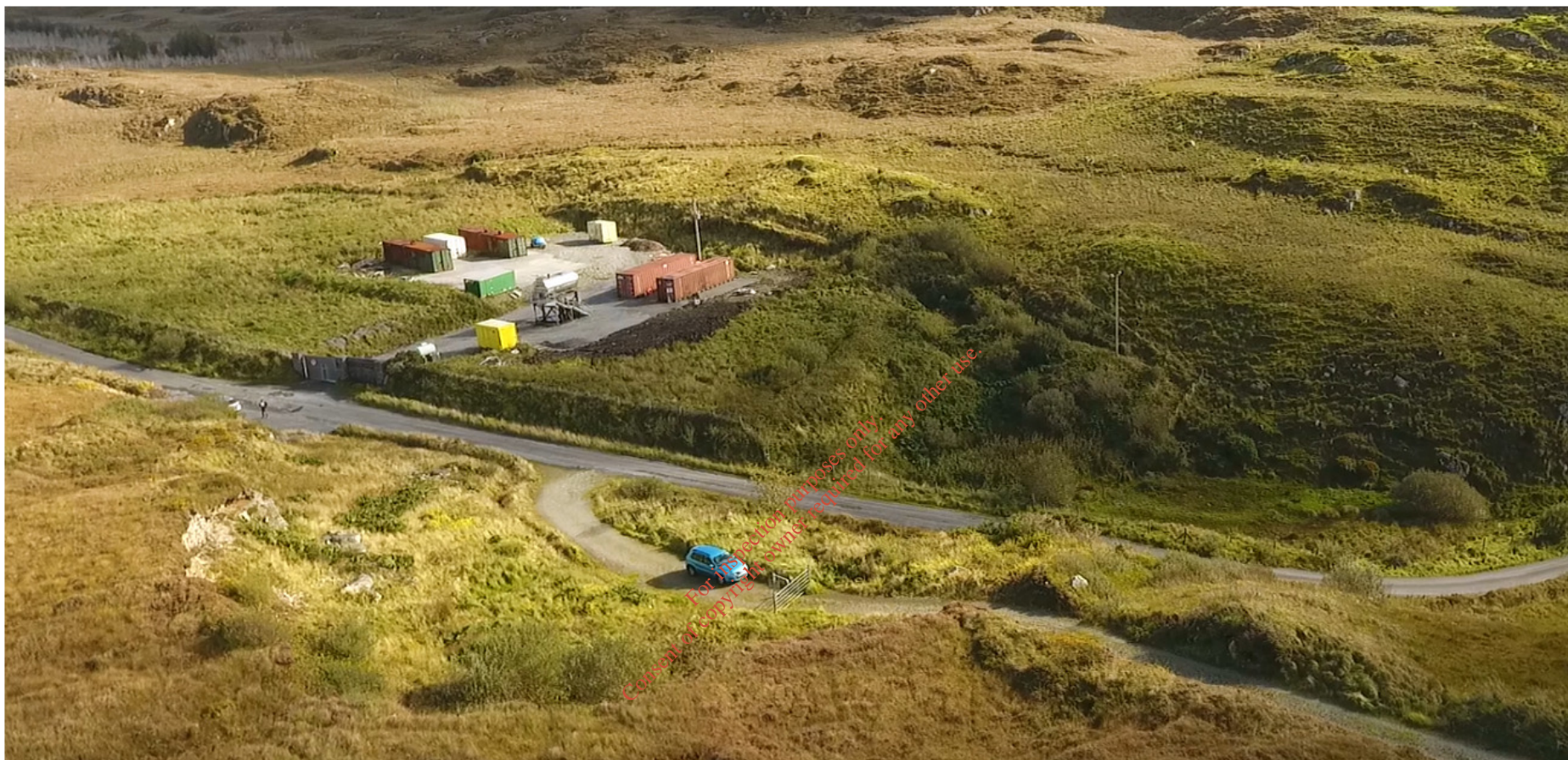
Plate C4.1. Aerial photograph taken on 29 th September, 2019 of Former Tullyvogheen Landfill taken at 30m elevation from the northwest of the site facing southwest showing Galway C.C. roads depot area to the west of the site and grassed/capped area to the middle and east of the site
