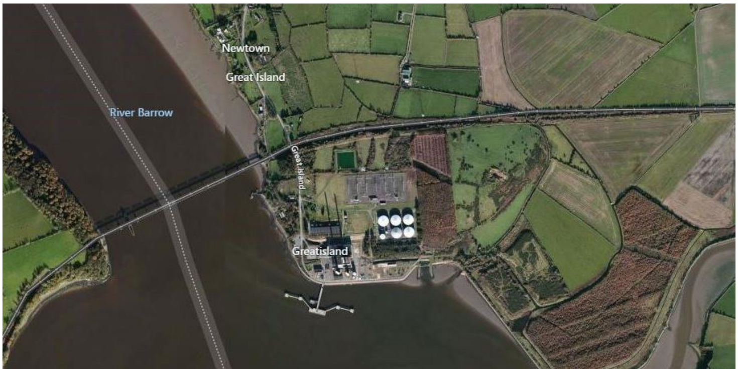
Figure 1: An aerial photograph showing the power station at Great Island, County Wexford.
