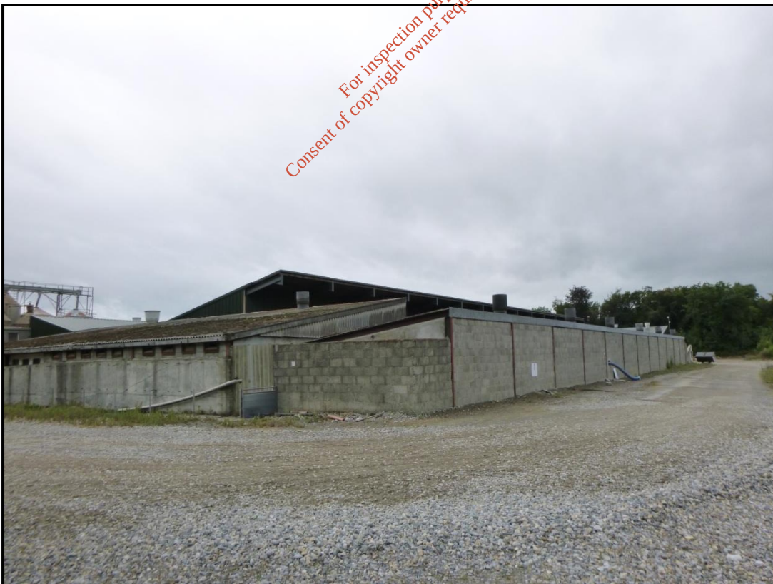
Plate 11.3: View to southwest from northeast corner showing buildings proposed for demolition (17th July 2019).
