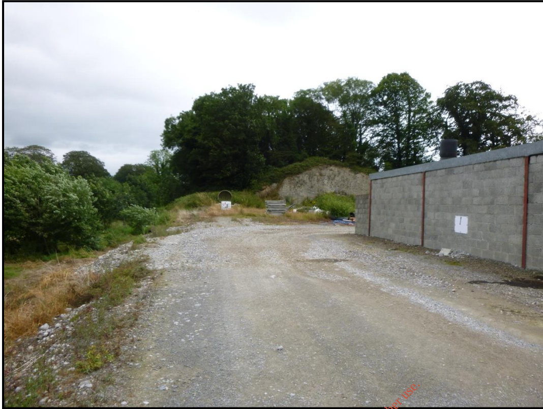
Plate 11.4: View to east from rear of the existing facility showing gravel platform formed by levelling a tree covered glacial till ridge evident in the centre background (17th July 2019).
