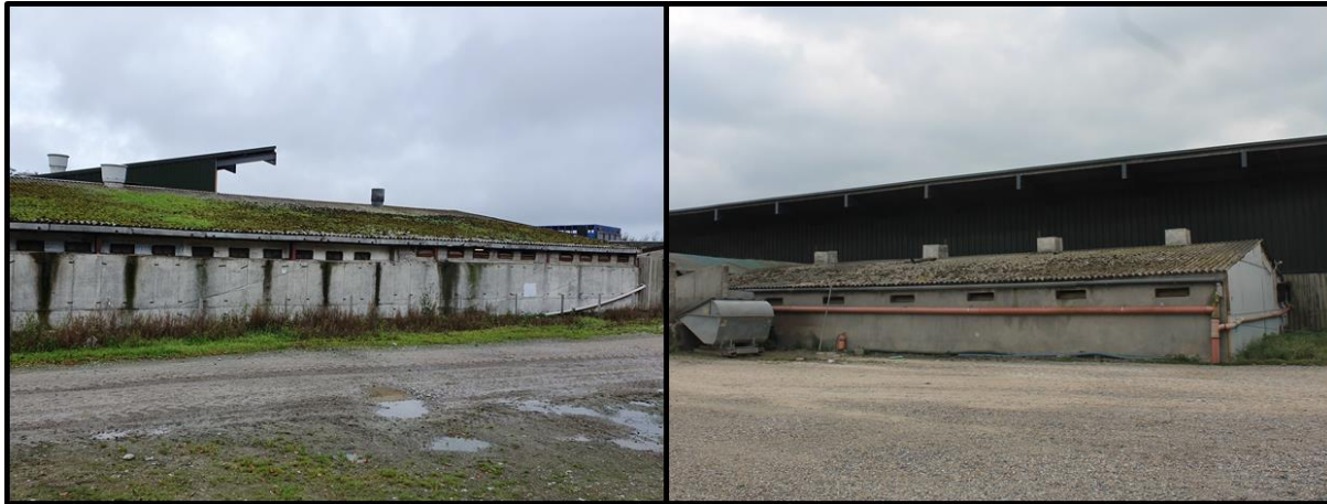
Figure 8.2: Buildings scheduled for removal.
