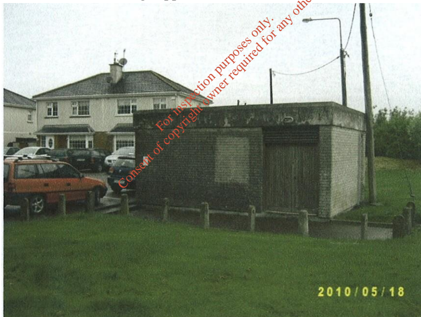
Existing pumping station viewed from the south.
