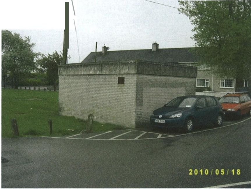
Existing pumping station viewed from the west.
