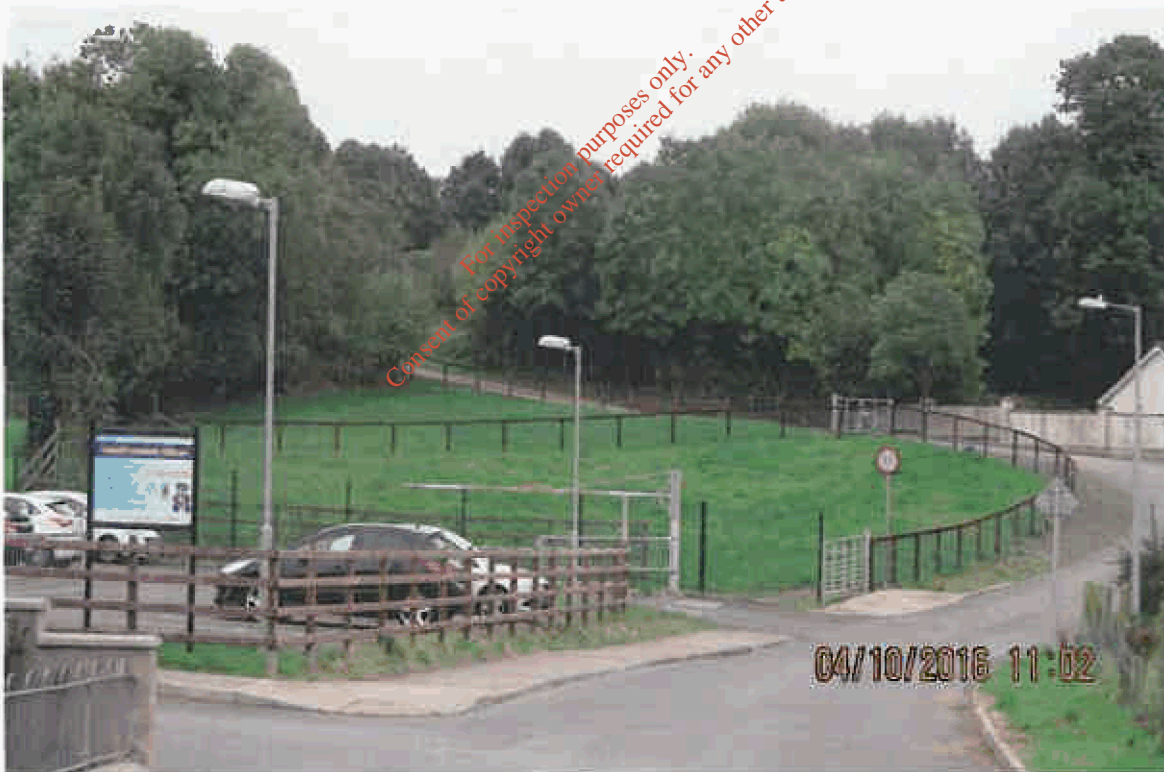
Photograph 2 Completed site viewed from Cootehill
