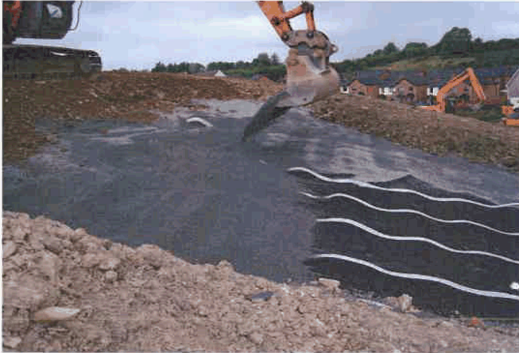
Photograph 9 showing capping layers.
