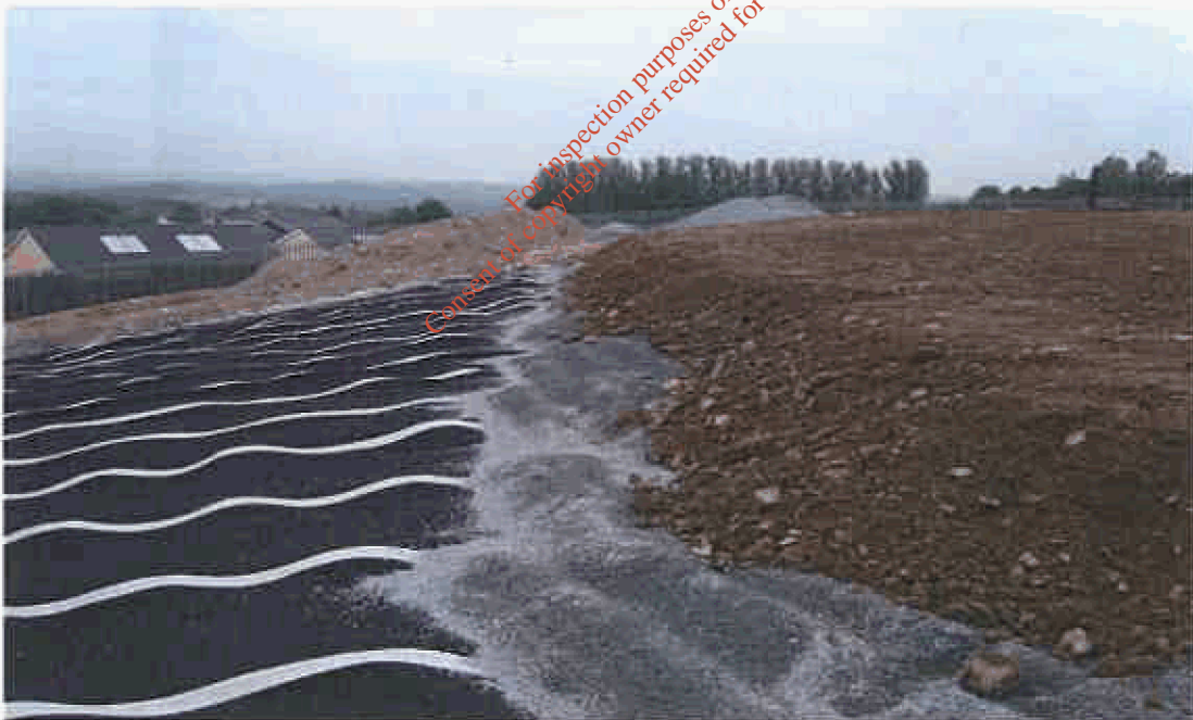
Photograph 8 showing placement of final layer of soil
