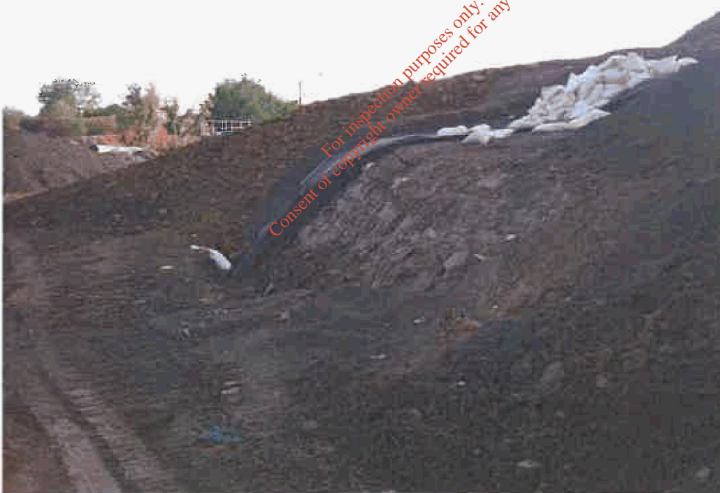
Photograph 10 showing anchor trench
