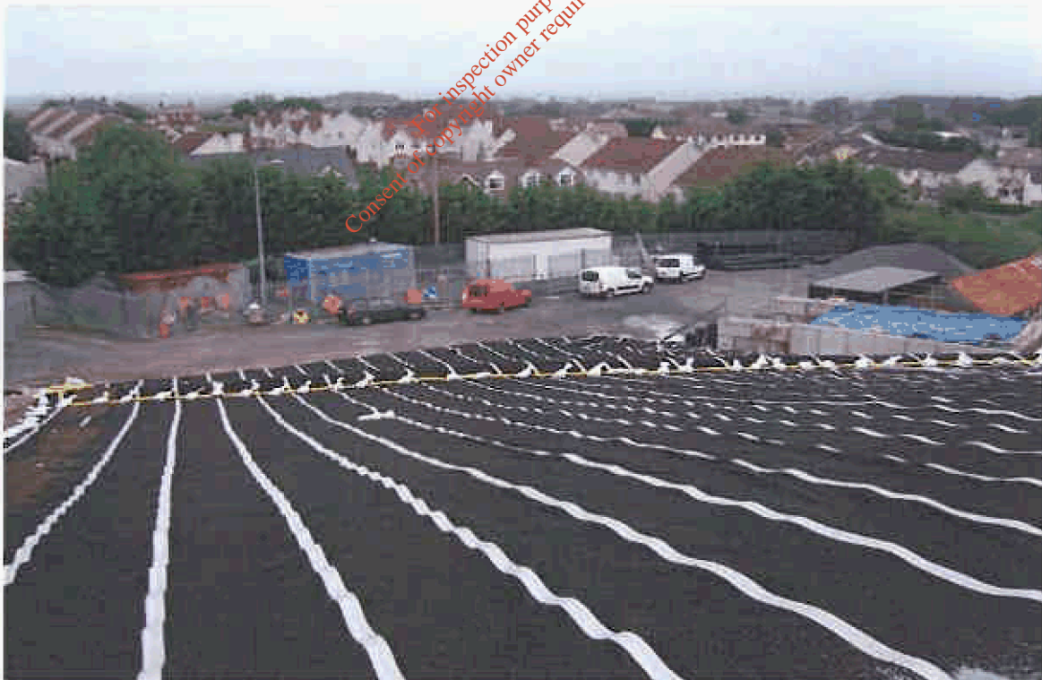
Photograph 6 showing LLDPE liner and surface water collection (yellow pipe).
