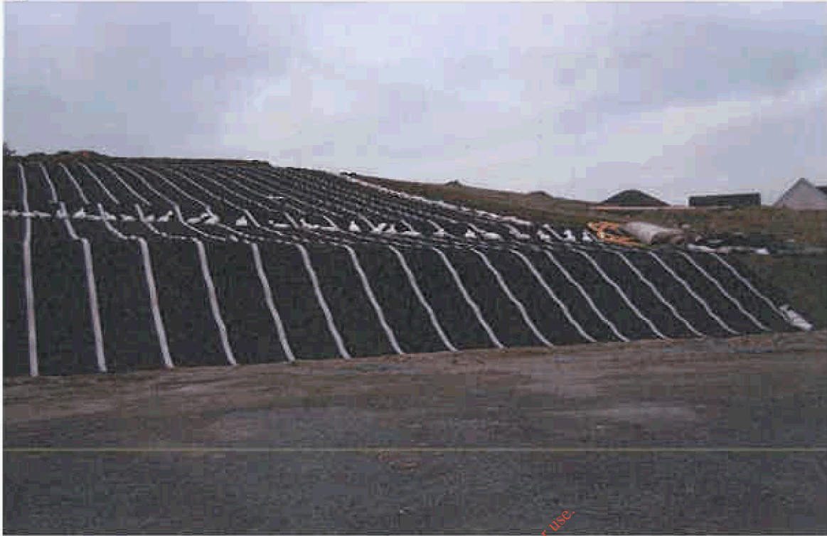
Photograph 5 showing the LLDPE liner being rolled out.
