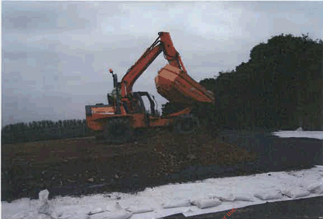
Photograph 7 showing Terram top layer in place covered by pea gravel in turn covered by the final soil cap.
