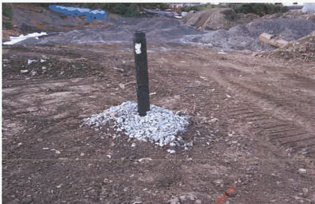
Photograph 13: Passive venting gas well
