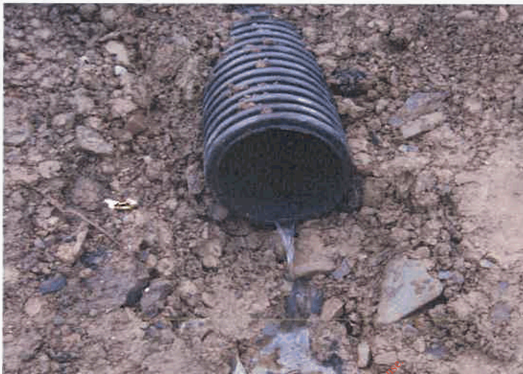
Photograph 12: Outflow from surface water collection system.
