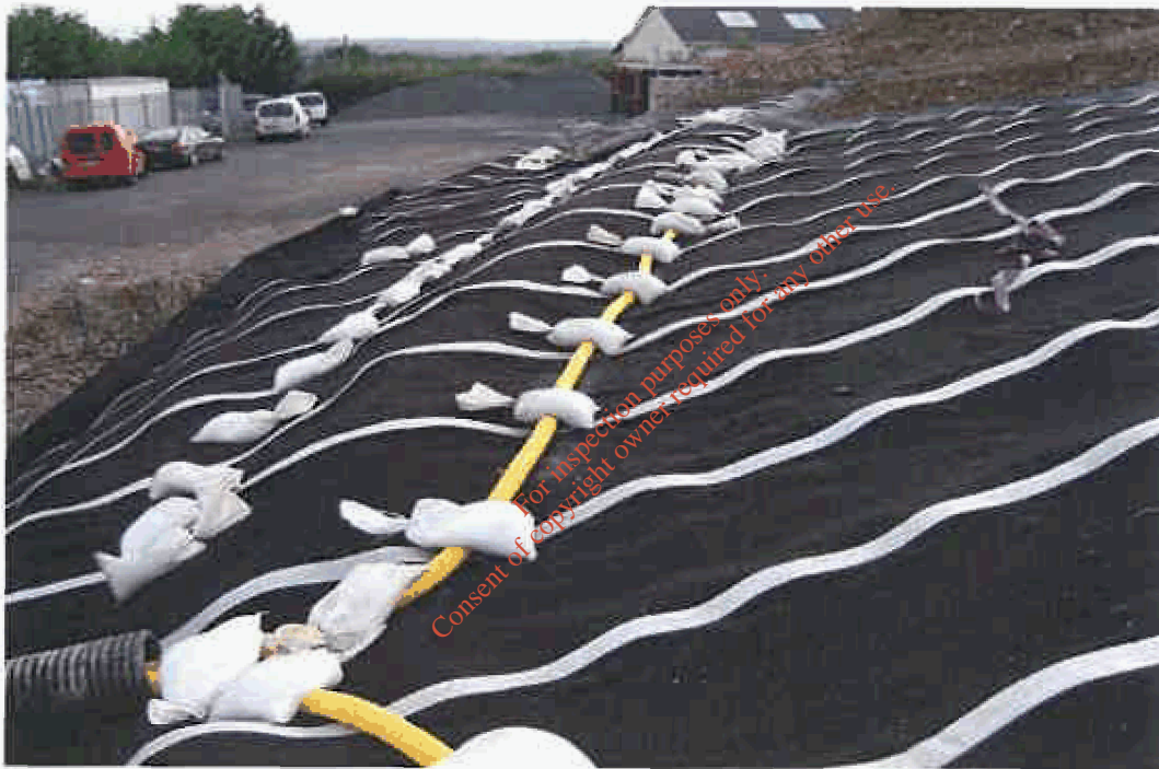
Photograph 11 showing slatted pipe (yellow) for collection of surface water running into larger (black) pipe.
