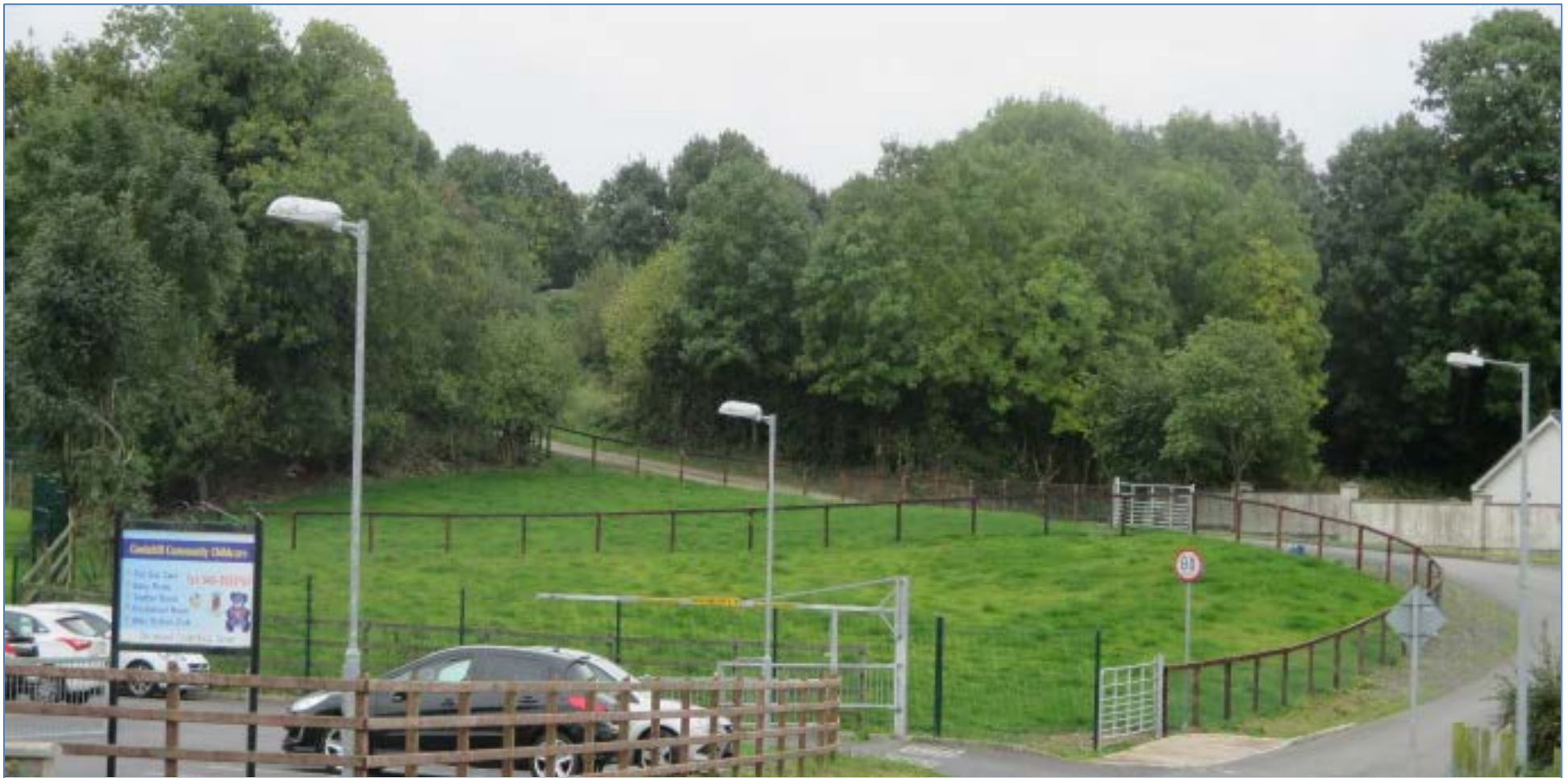
Figure 3: Current condition of the landfill site
