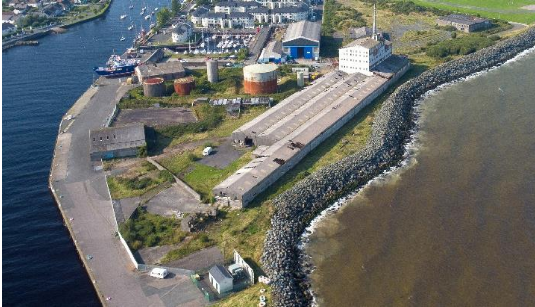
Figure 13.19: Old Wallboard facility and other industrial structures at Ferrybank
