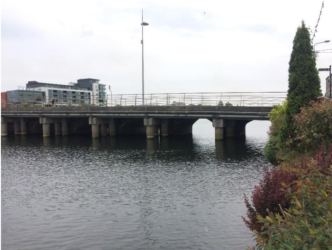
Figure 12.9: Arklow Bridge (RPS A26), facing east-southeast
