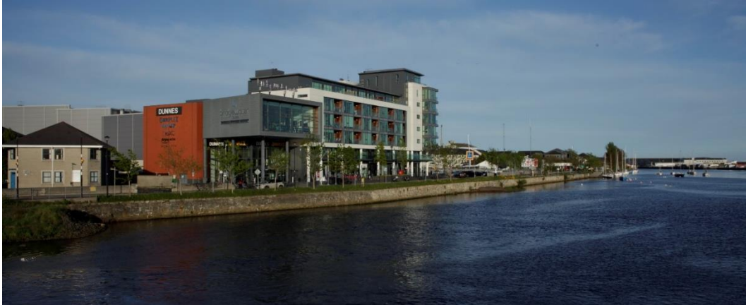
Figure 13.15: North Quay and Bridgewater Shopping Centre from Arklow Bridge
