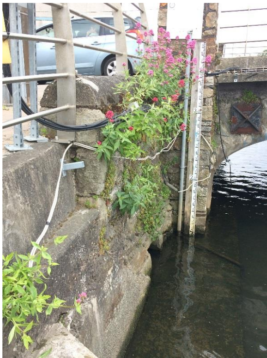
Figure 12.11: Wall abutting the south-eastern side of Arklow Bridge, facing northwest
