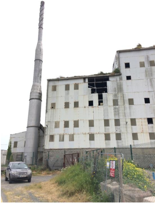
Figure 12.17: Existing factory structure within the WwTP site, facing northeast
