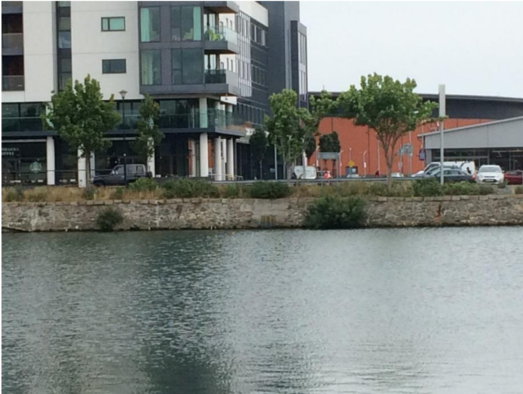
Figure 12.14: Section of the rubble North Quay wall, facing northeast
