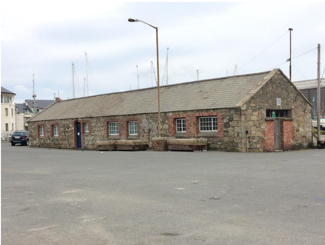
Figure 12.16: Early 19th century Salvage Store, facing north
