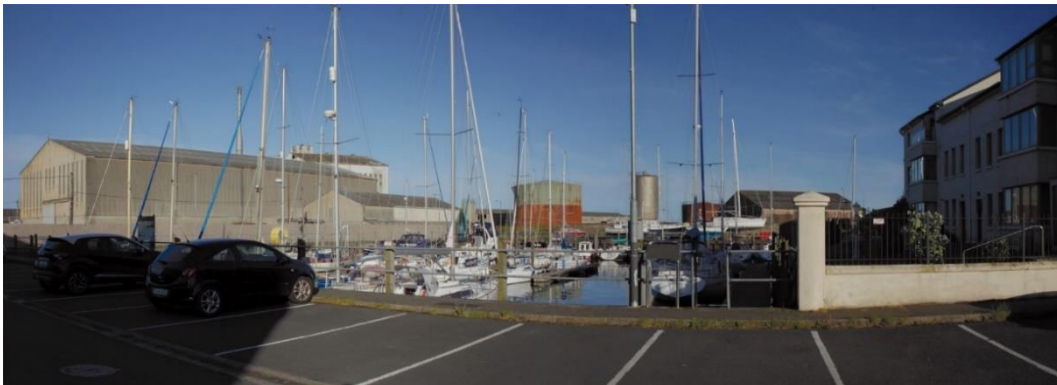
Figure 13.18: View from Marina Village across Arklow Marina in the foreground and to industrial buildings beyond
