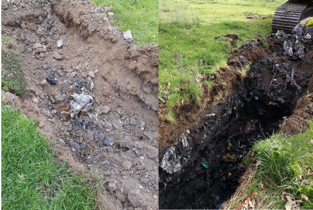
Plate 3.2 Trial Pit excavation
