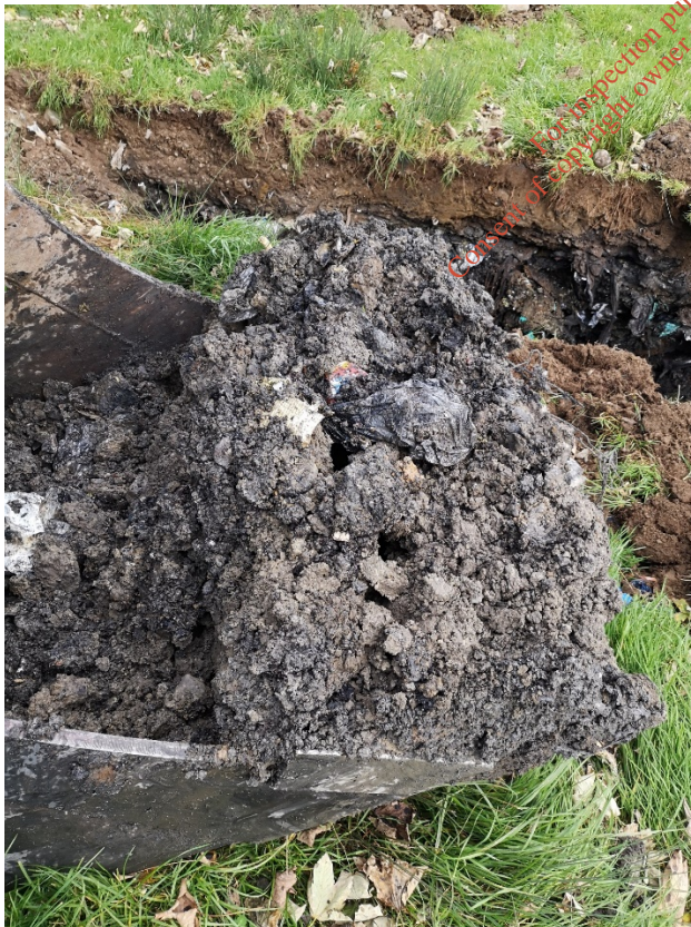
Plate 3.3 Trial Pit material extracted
