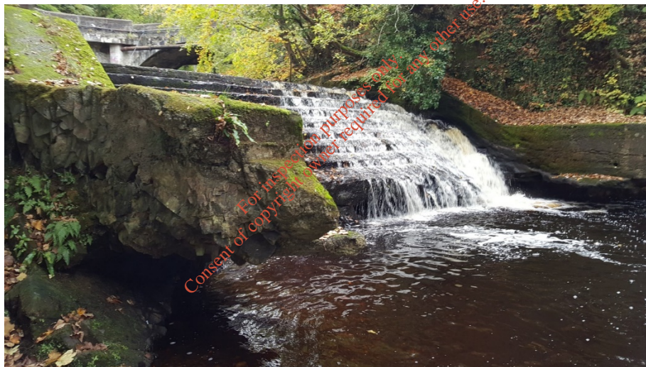
Plate 2.3 Bridge apron upgradient of the site
