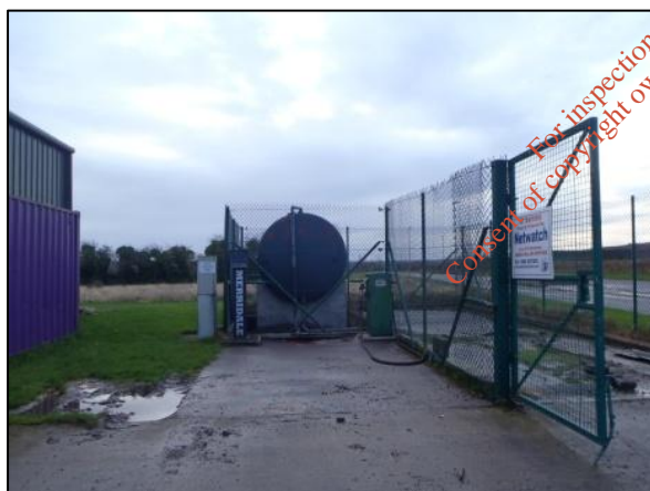
Plate 8 – Diesel Storage Tank
