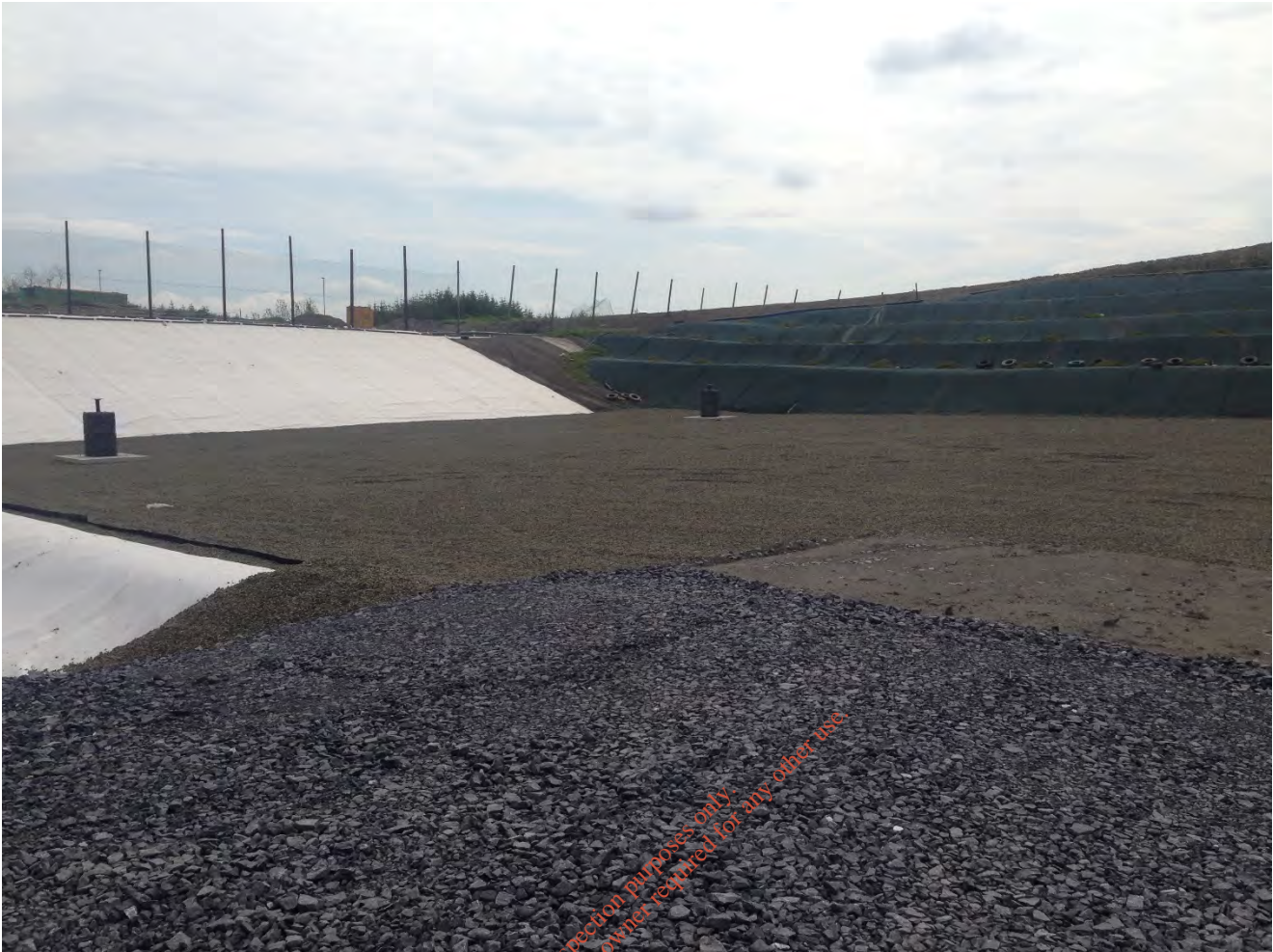
Plate 2-3: Lined cells at Knockharley Landfill
