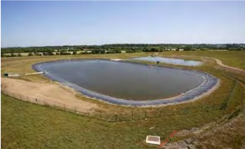
Plate 2-5: Surface Water Attenuation Pond and Wetland
