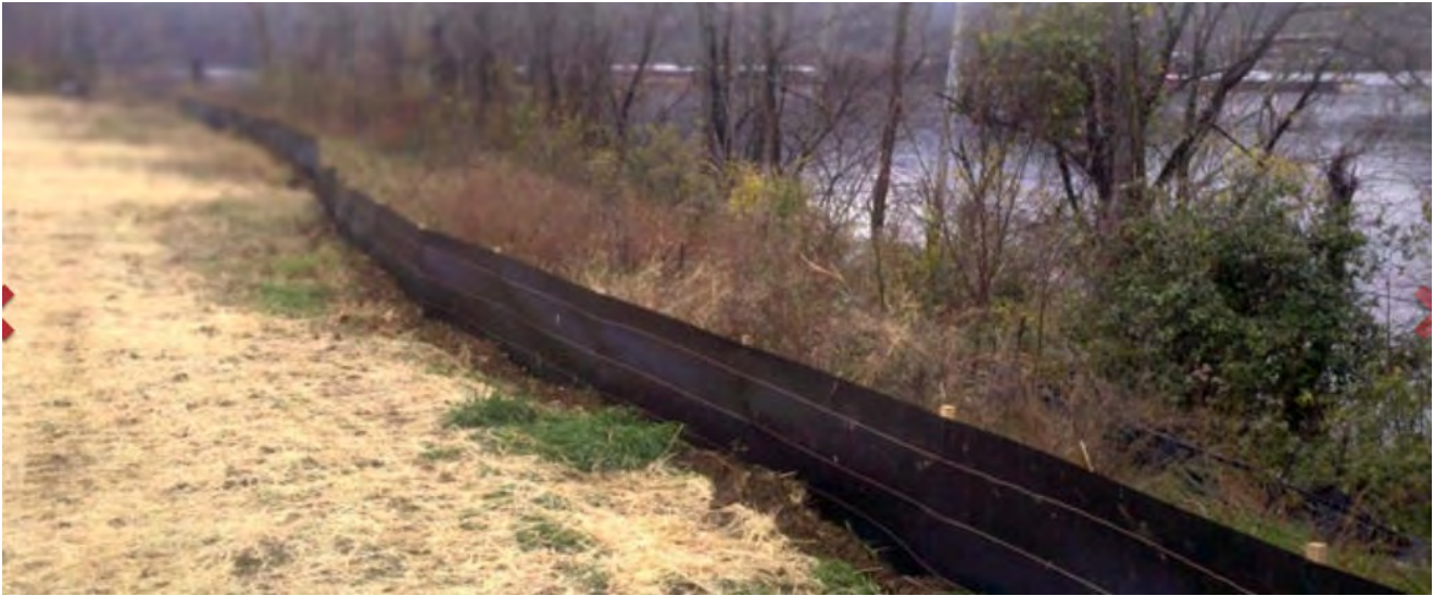
Figure 4.4: Typical Silt Fence 2
