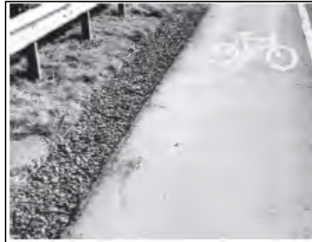
Figure 4.3: Typical Filter Drain
