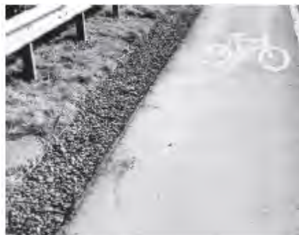
Figure 2.5: Typical Filter Drain
