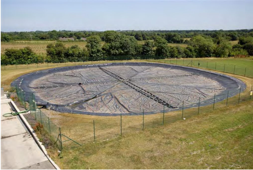
Plate 2-4: Covered Leachate Lagoon
