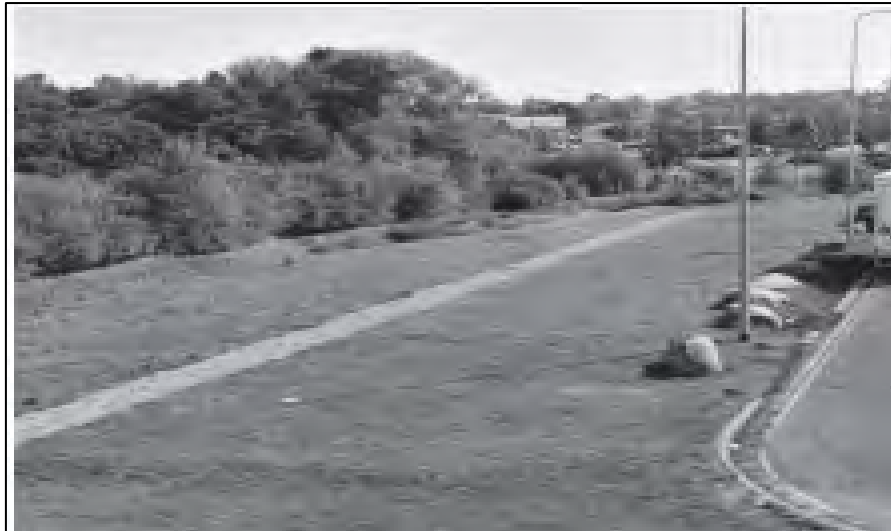
Figure 4.1: Typical Filter Strip
