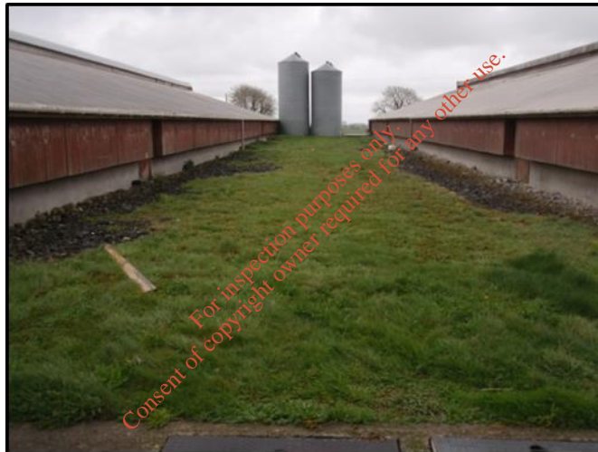
Plate 16.4: Looking E between House Nos. 11 & 12.
