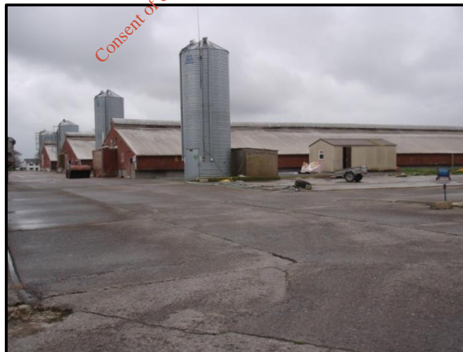
Plate 16.2: Looking SSW across site showing House Nos. 10, 11 & 12.
