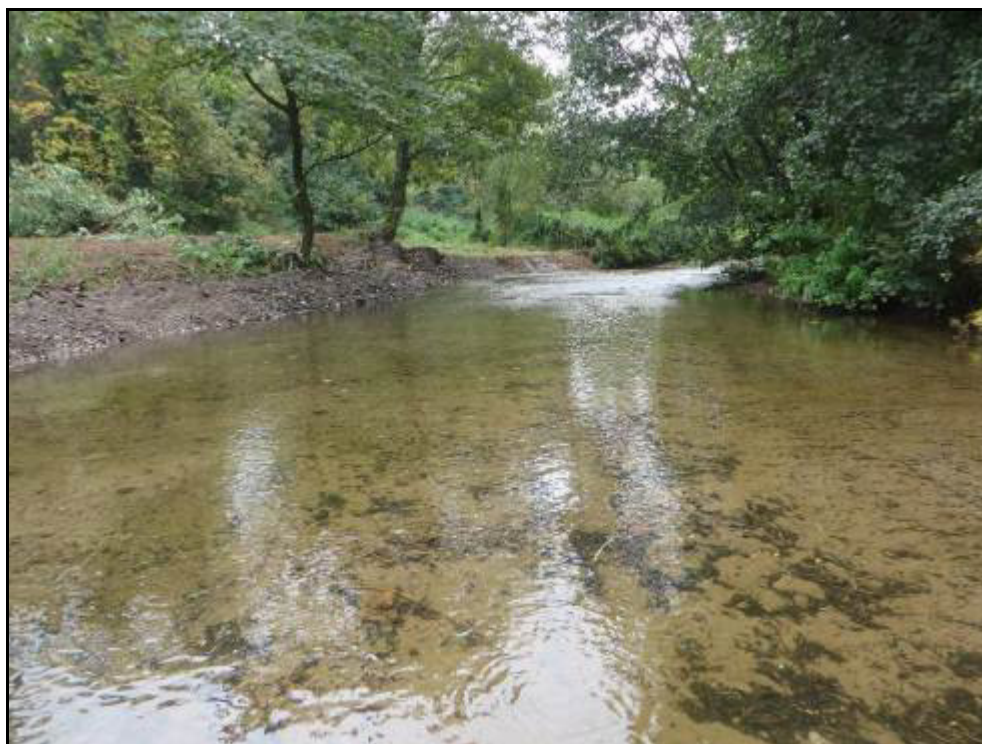
Plate 30 The stretch of the River Finnow affected by instream works has been widened and the substrate was found to be covered in a layer of silt during the current assessment.
