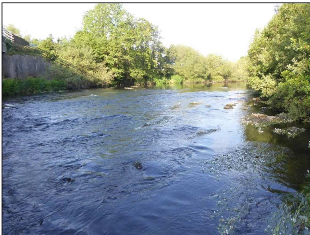
Plate 1 Site 1 was located at Keale Bridge (R583) on the Blackwater River.
