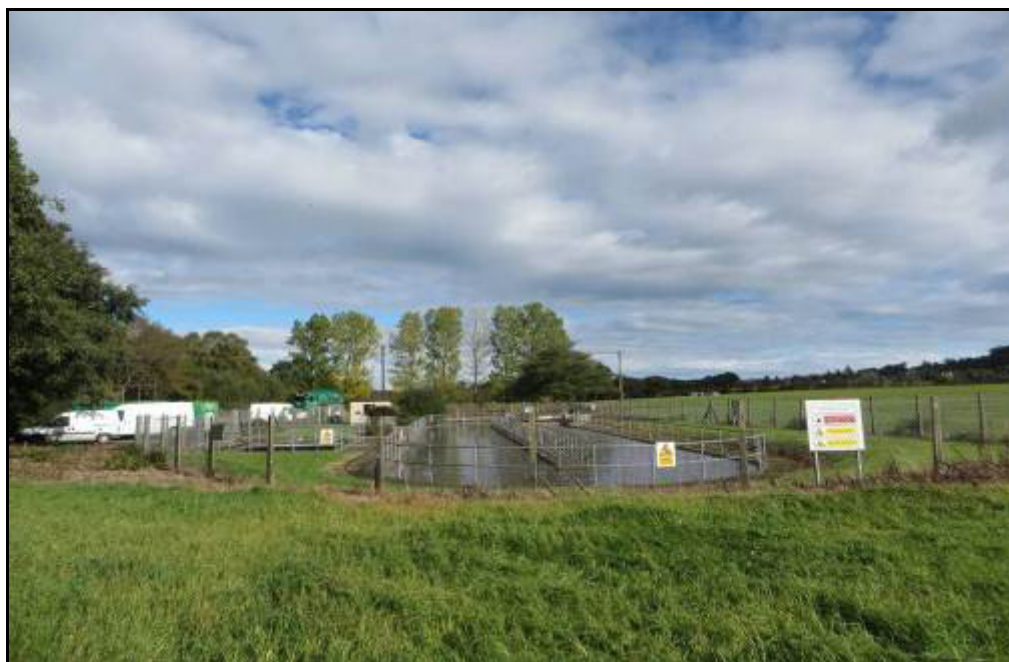
Plate 1 The existing Millstreet Sewage Treatment Plant.
