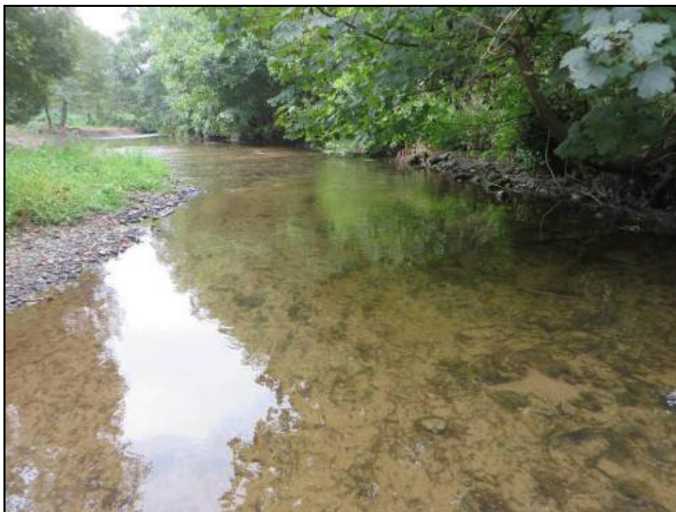
Plate 33 River Finnow downstream of the instream works area after the water had cleared. A significant layer of silt had been deposited on the riverbed from the works area to the River Blackwater.
