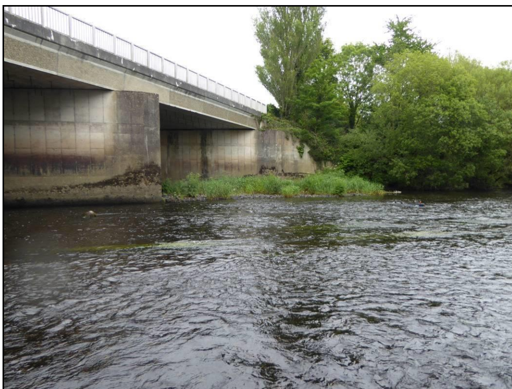
Plate 48 Transect 14 - 4 FPM: 3 alongside right bank + 1 mid channel.
