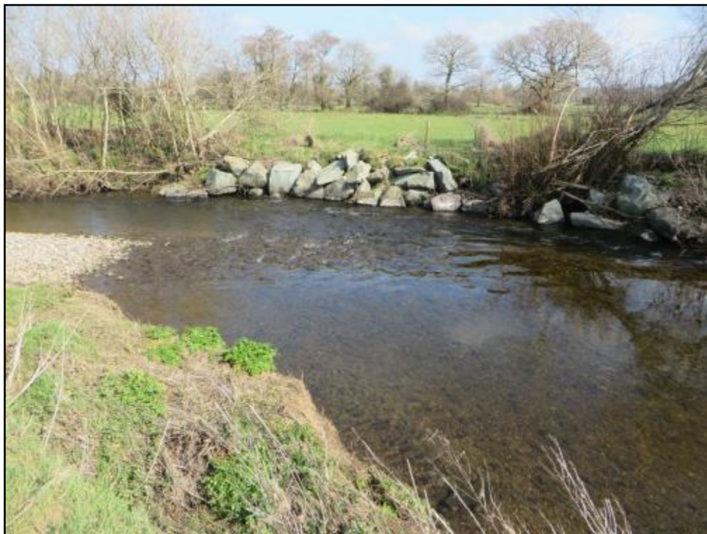
Plate 15 Bank erosion was constant feature throughout the length of the surveyed stretch. Bank reinforcement works are shown above.
