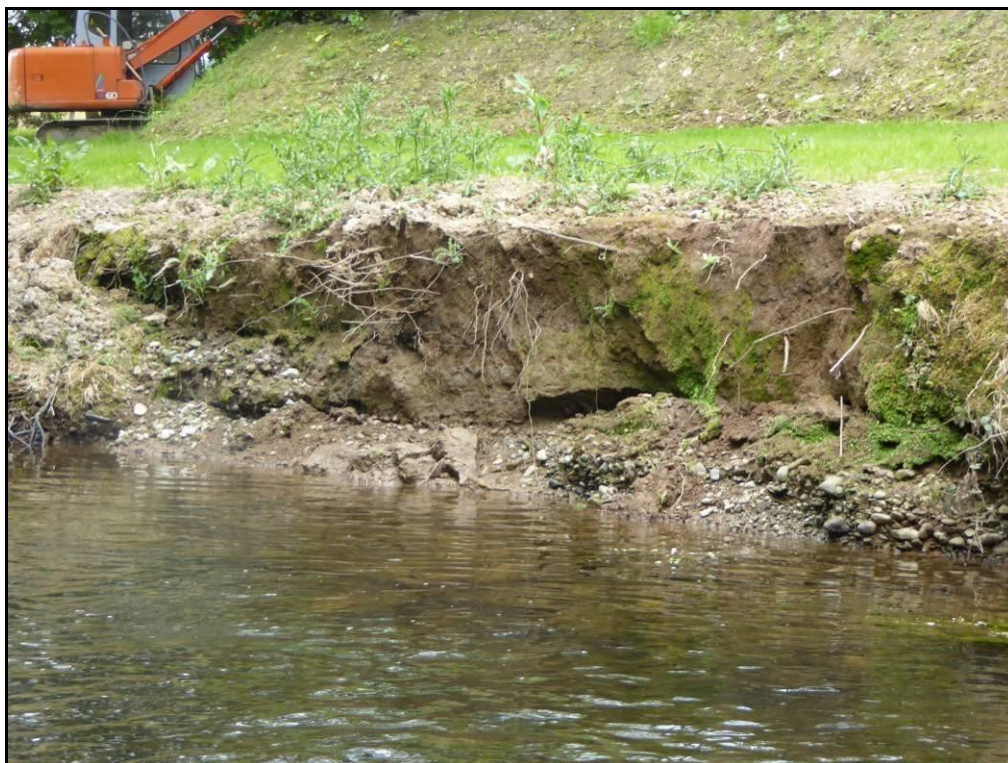
Plate 55 Bank erosion on River Finnow within the grounds of Drishane Castle following instream works carried out in 2014.
