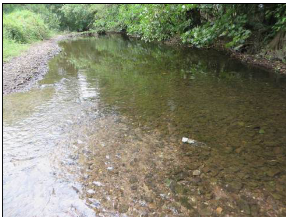
Plate 32 Upper limit of the instream works was obvious from the change in substrate conditions.
