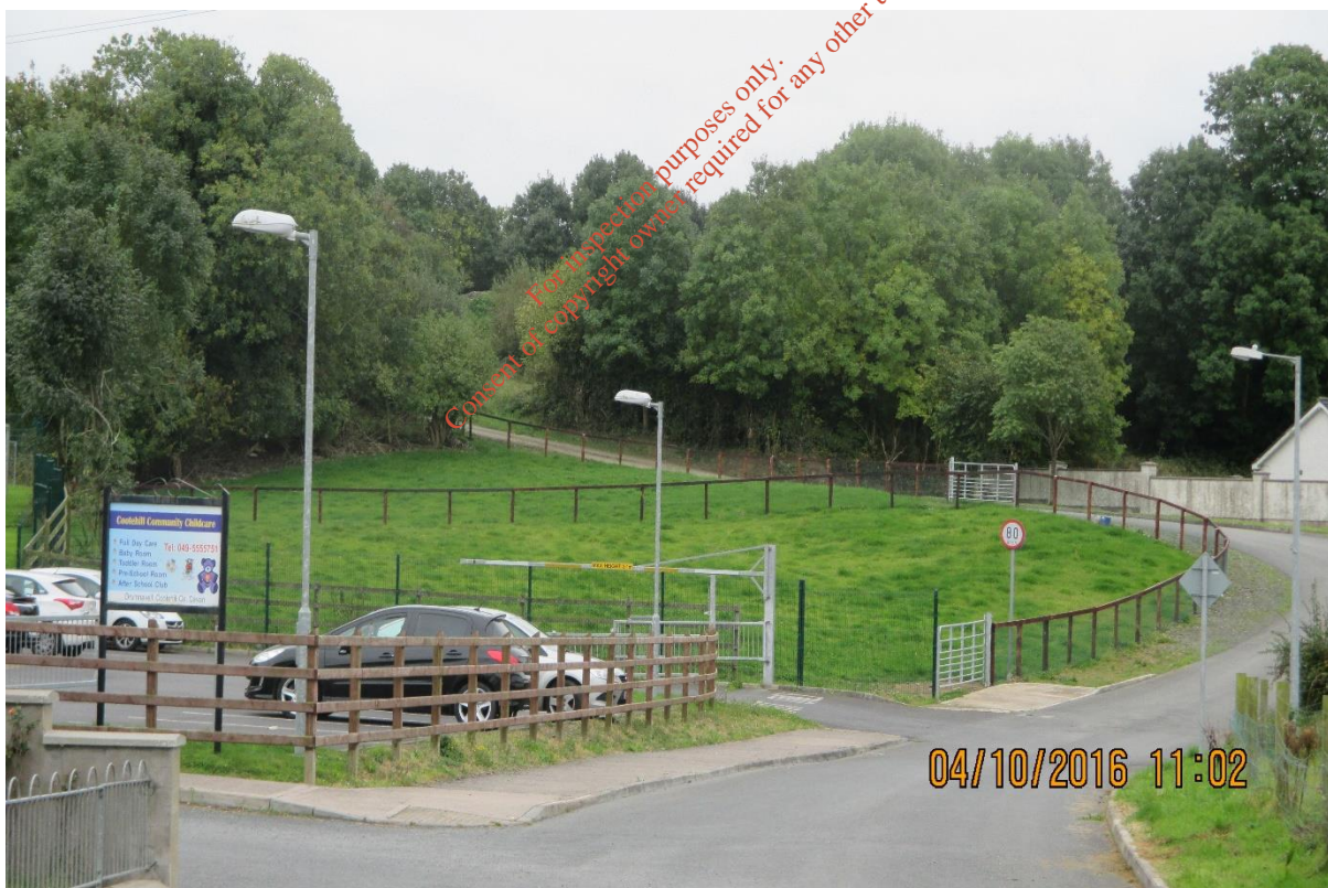
Photograph 2 Completed site viewed from Cootehill
