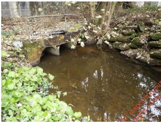
Stream at downstream end of triple culvert under R576
