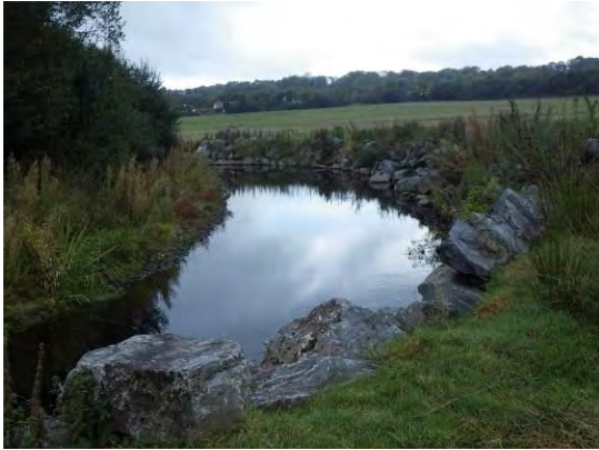
Section of reinforced bank
