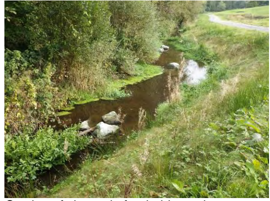
Section of channel after habitat enhancement diversification works
