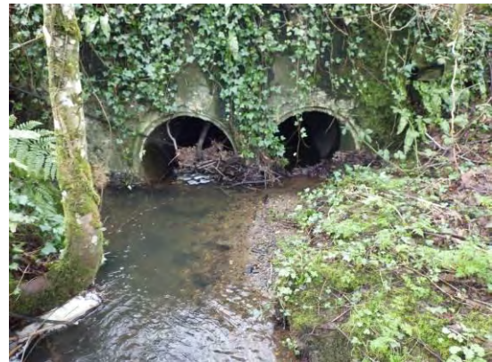
Twin culvert at Park Bridge
