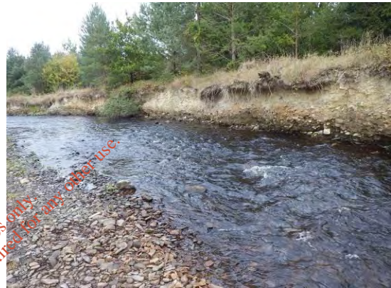
Severely eroding river bank
