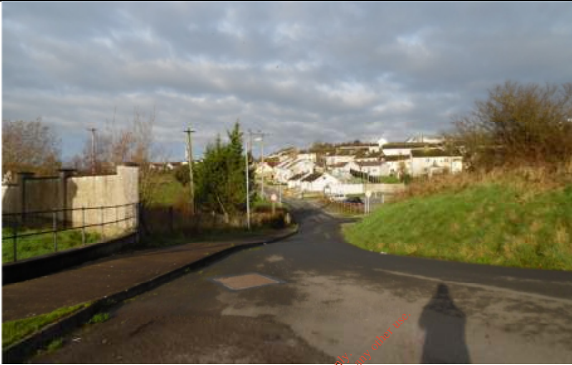
Photograph 1 : Location No 1 - Eircom Service Duct outside the southern Boundary.
