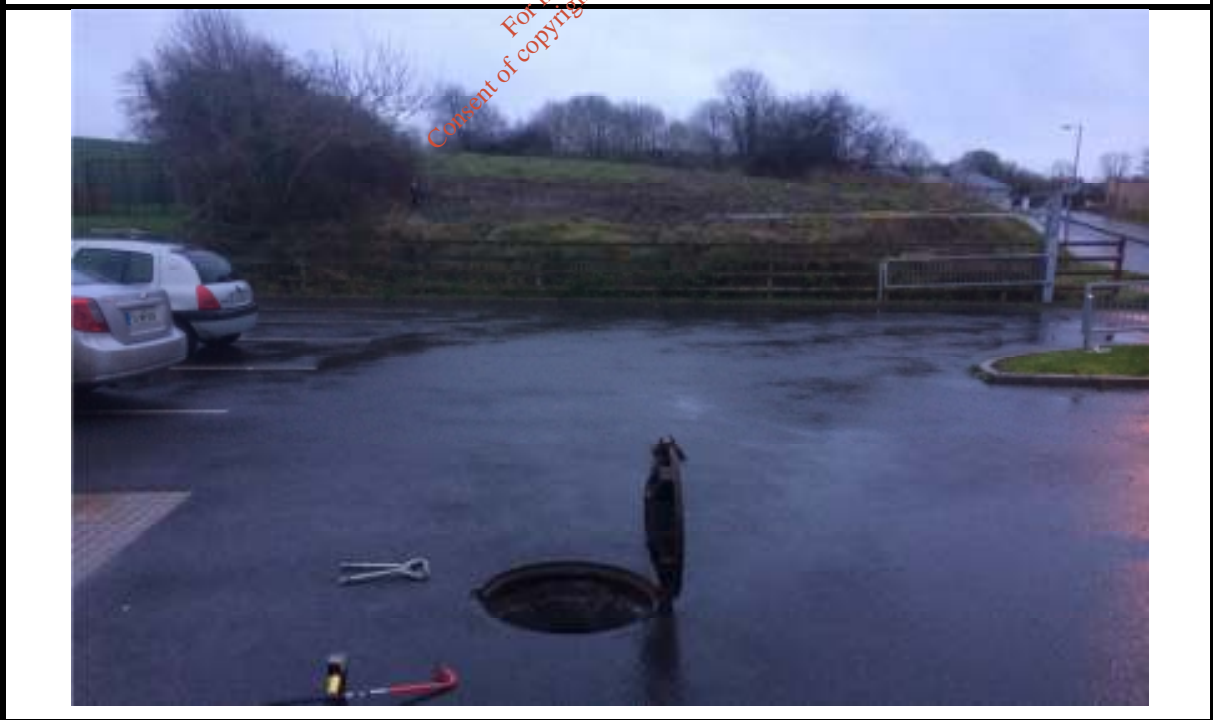
Photograph 4: Location No. 4 Inspection Manhole for Foul water.
