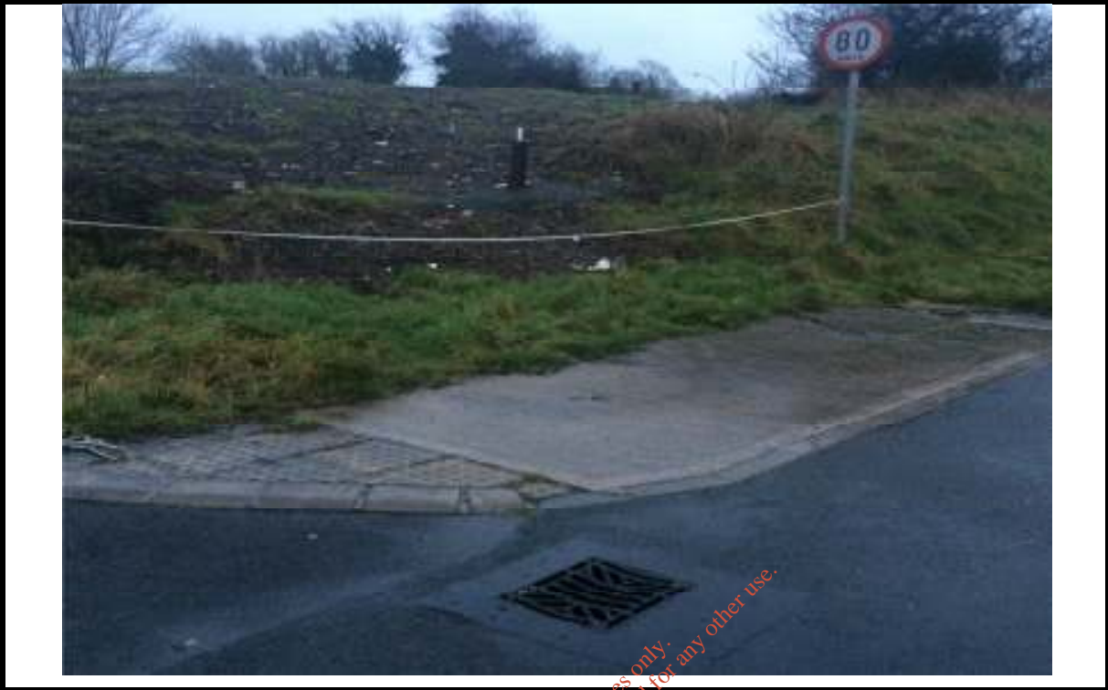
Photograph 3: Location No. 3 Surface Water Road Gully outside the Westerly Boundary.
