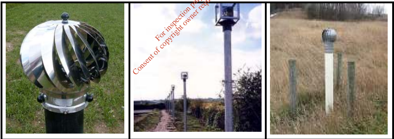
Figure No. 6 Rotating Aspiromatic Cowl
