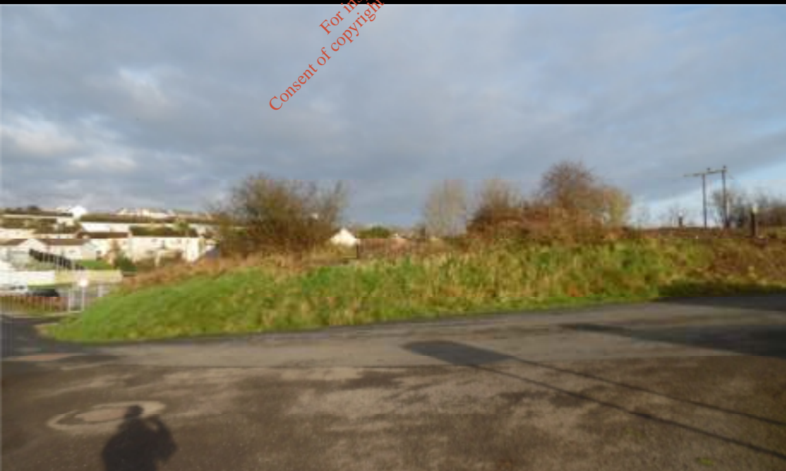
Photograph 2: Location No. 2 Eircom Service Duct outside the southern Boundary.
